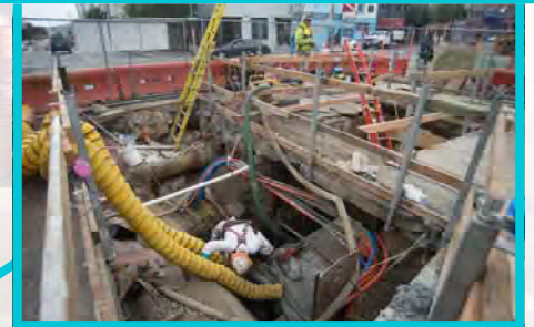
4th St. Surface Track, Systems (STS)
