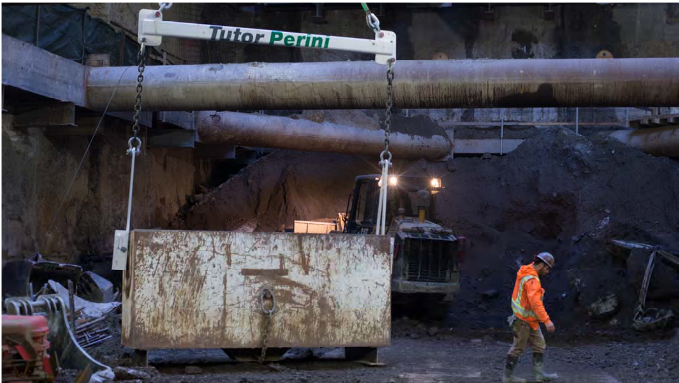
A worker coordinates with a bulldozer at the bottom of the headhouse to offload soil excavated from the cross-cut cavern and station cavern.
