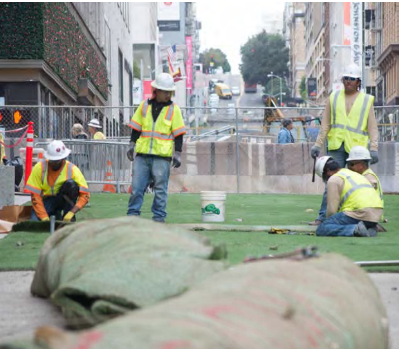
2 Green turf, lighting, and seating are installed
