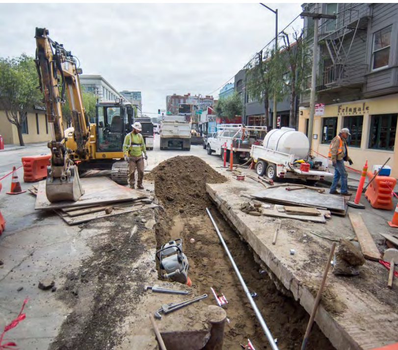
2 A trench is dug and utilities are installed or upgraded
