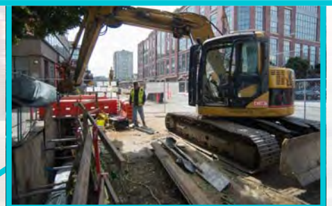
4th St. Surface Track, Systems (STS)
