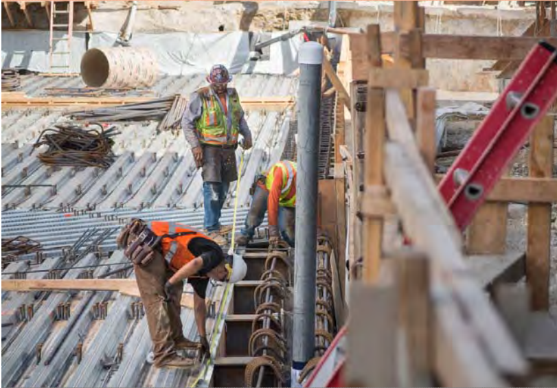
1 Installation of deck panels over steel and reinforced concrete structural elements
