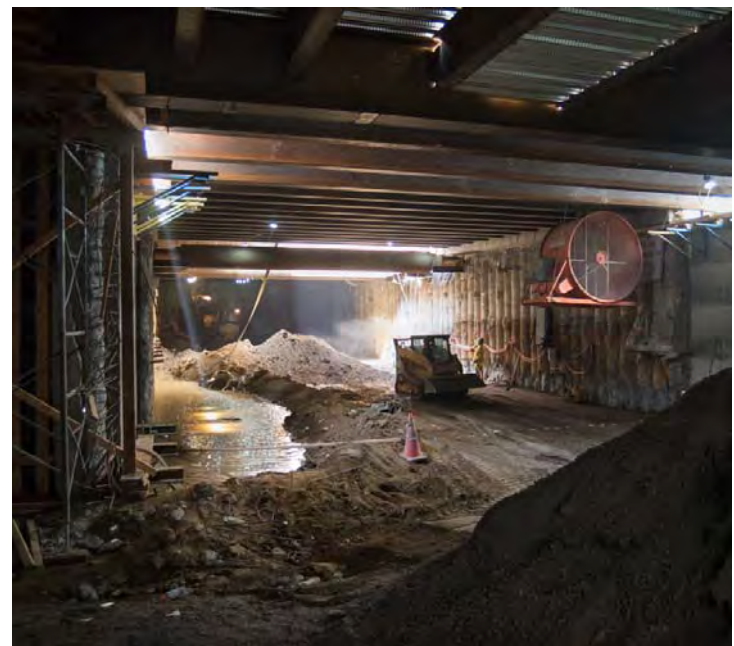
3 Excavation of the concourse interior continues underground
