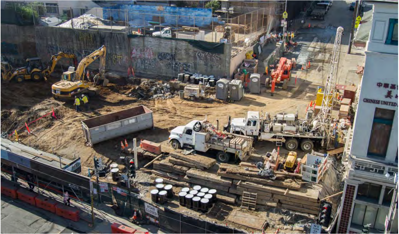
With underground wall construction complete, site demobilization is underway.
