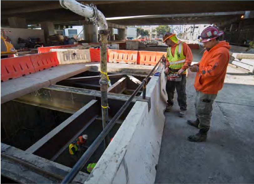
1 Work to construct the tunnel portal continues underground
