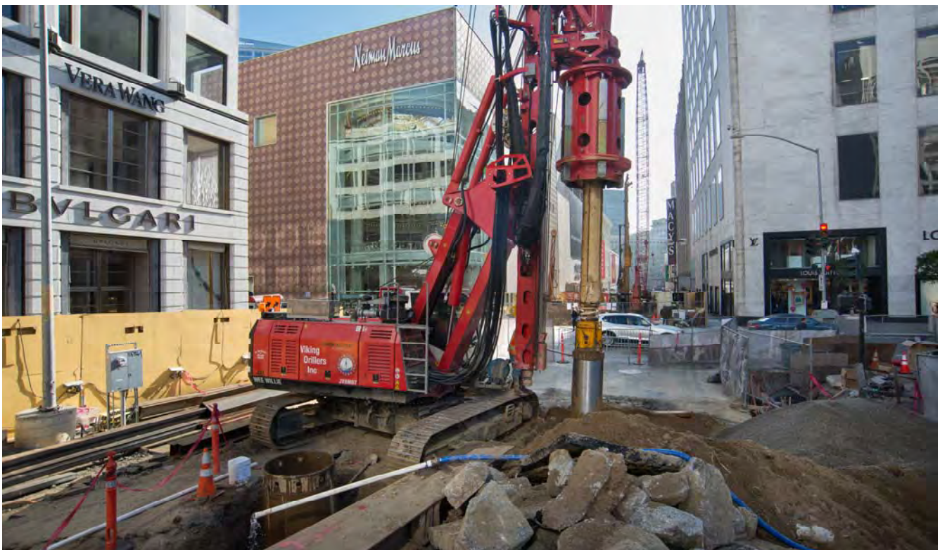
Underground wall piles are being installed on Stockton north of Geary.
