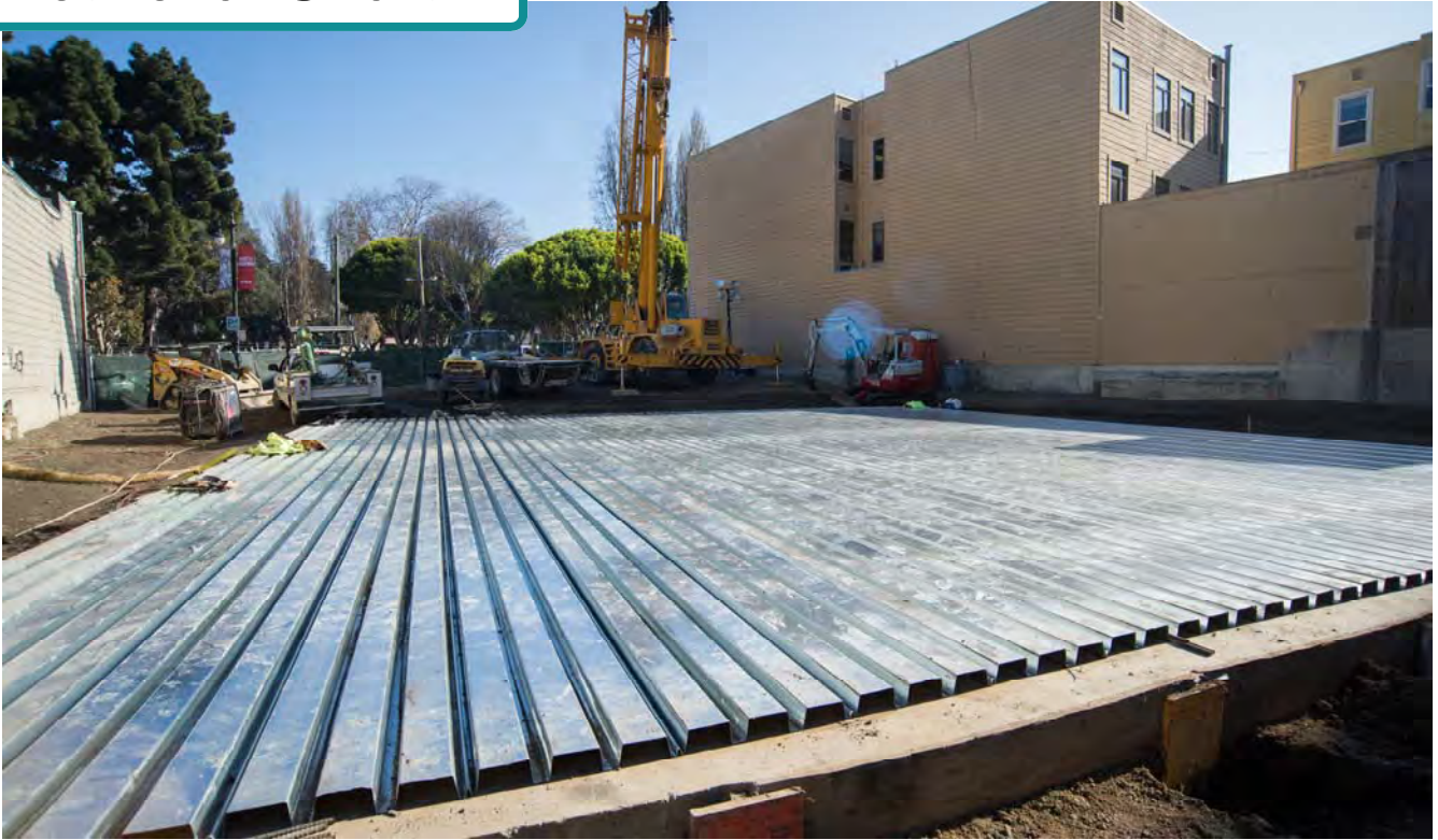
The TBM retrieval shaft has been decked over.
