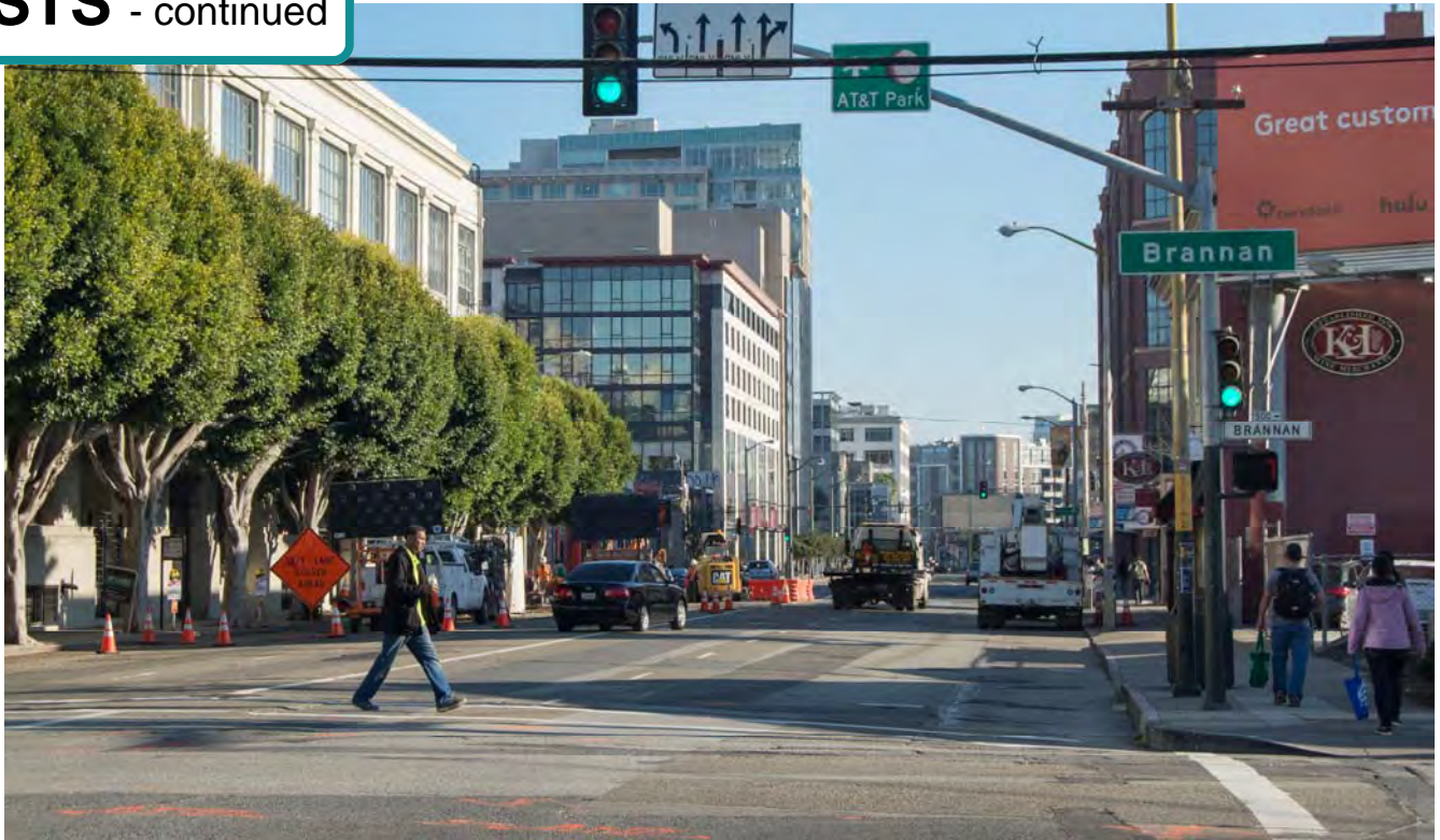
Utility work on 4th near Bluxome, south of Brannan, is ongoing.
