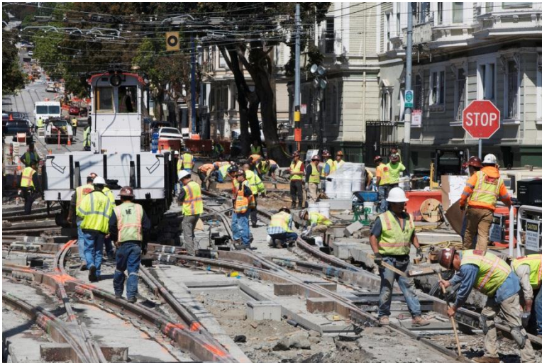
Figure 3: Rail Replacement at Church and Duboce streets
