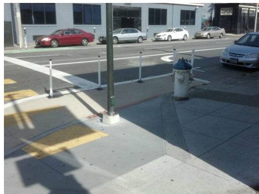
Image 4: Example of Painted Safety Zone
