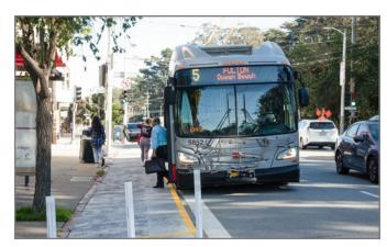
Temporary transit bulb on Fulton Street: Quick-build transit bulbs made of wood were installed on Fulton Street at 6th and 8th avenues. These will soon be replaced by concrete bulbs.
