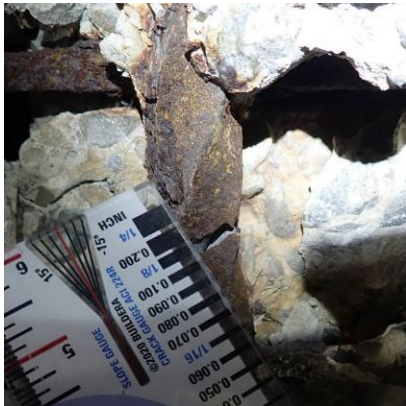
✕ 09+65 – Fractured Bar
