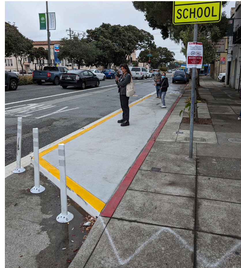
New widened sidewalk on Geary at 25th Ave inbound bus stop
