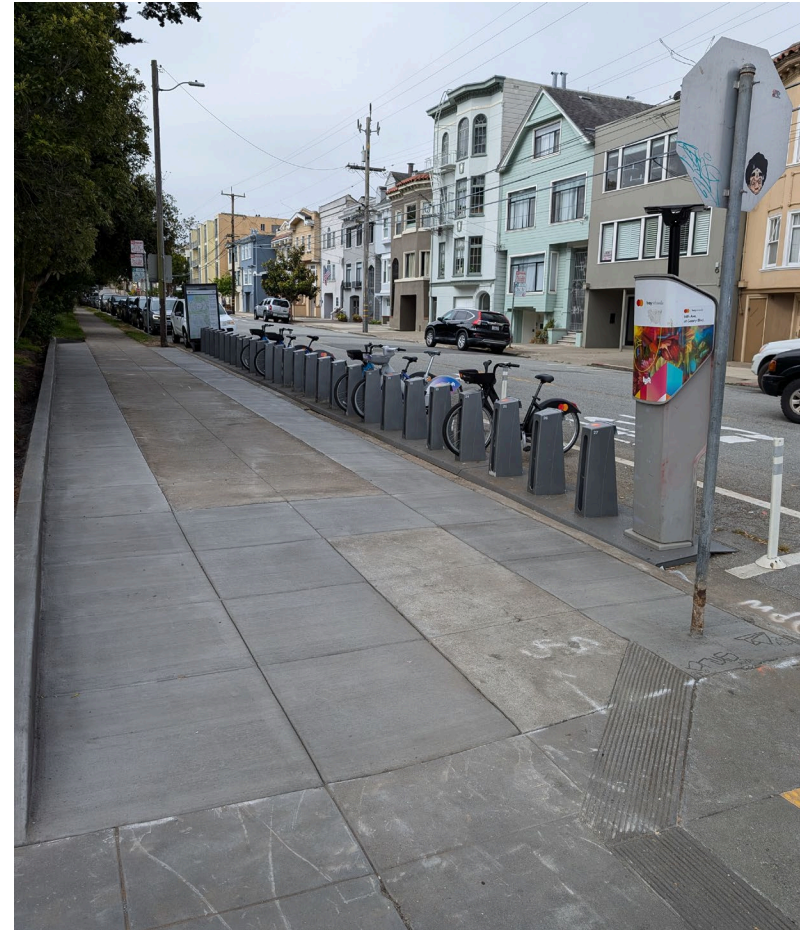
New widened sidewalk on 14th Ave south of Geary, before bike share station relocation
