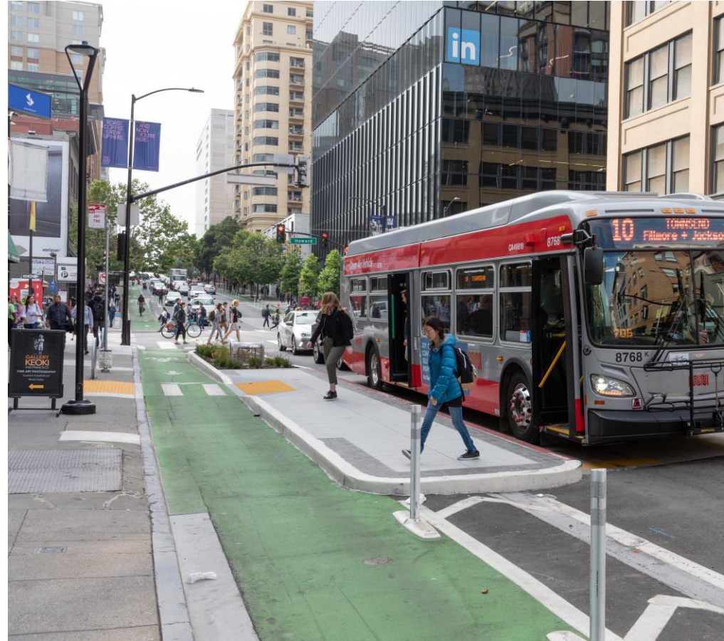
Example of a transit boarding island and protected bikeway (2 nd Street).
