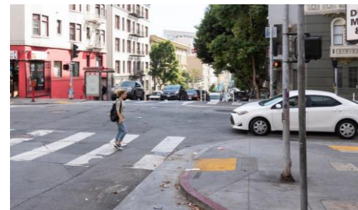
Sidewalk corner bulbouts
