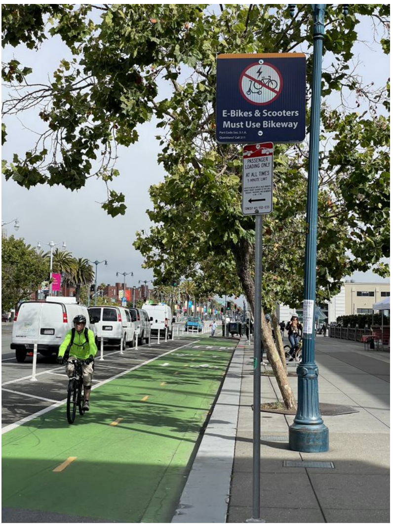
Example of a parking-protected bikeway on The Embarcadero with painted pedestrian access aisle
