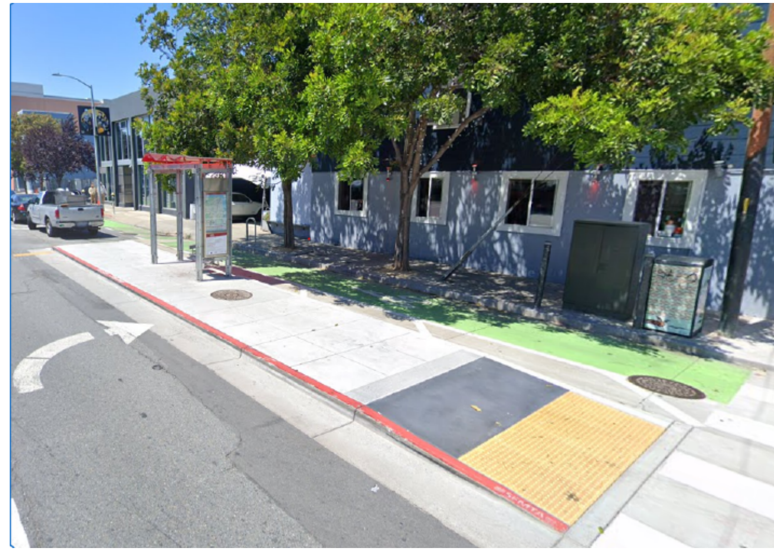
Example of a bus boarding island with protected bikeway in the SOMA neighborhood. Boarding islands allow for level, in-lane dropoffs and pickups and shorter crossing distances.
