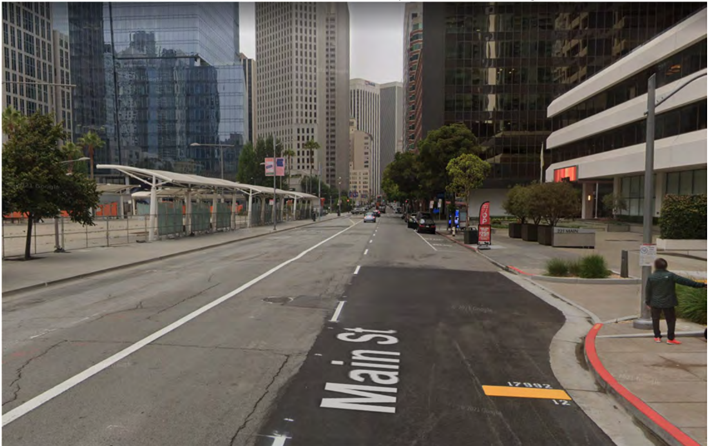
Main Street, midblock between Folsom Street and Howard Street, by Private Street, looking north
