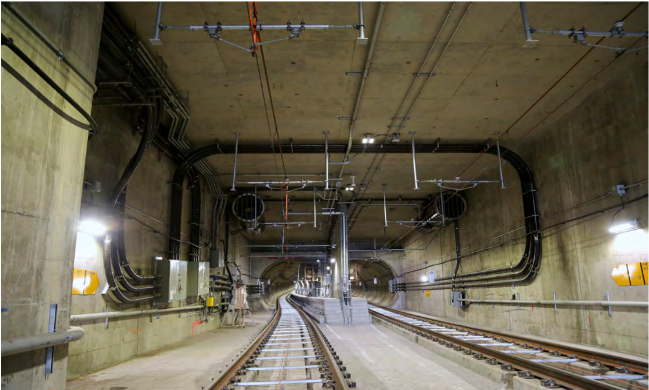
View of the portal entrance into the tunnel
