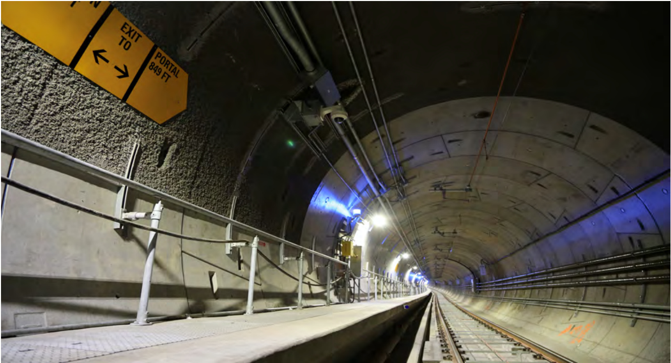
View from inside the tunnels
