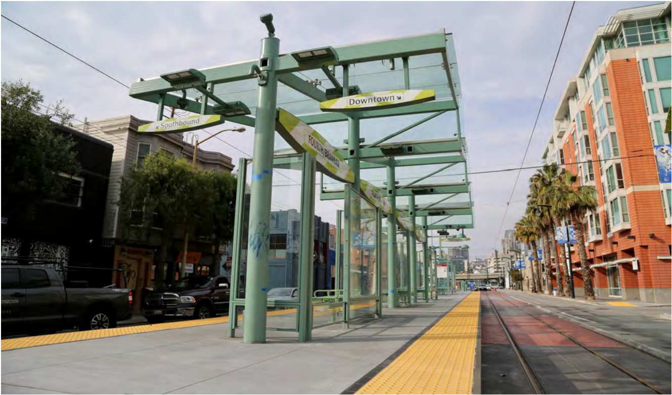
View of the platform at 4th and Brannan
