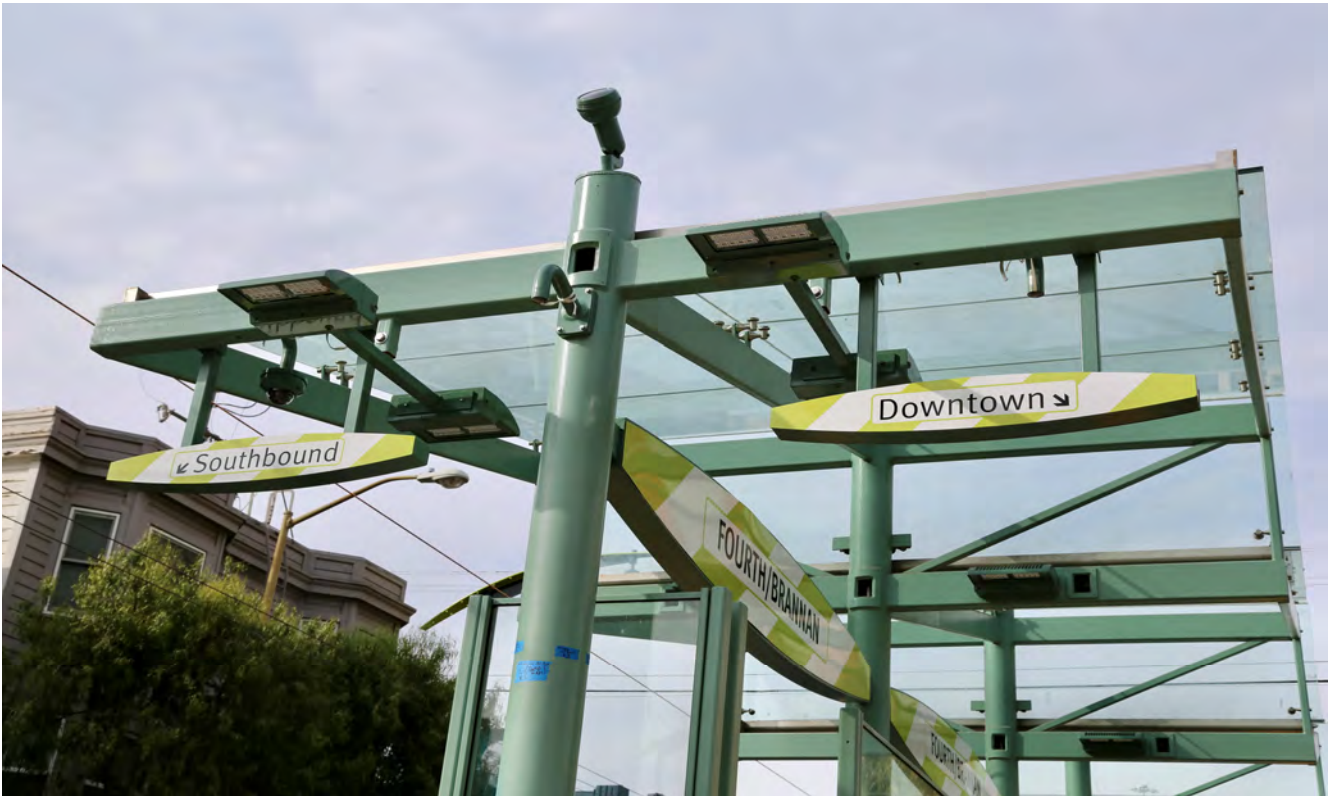
View of signage for STS Platform
