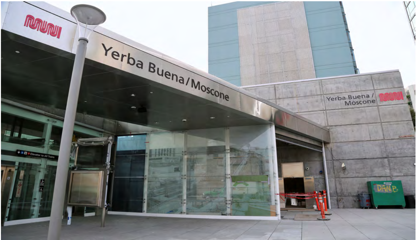
YB Entrance with signage
