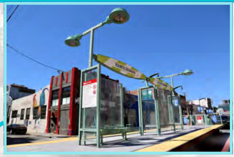
4th St. Surface Track, Systems (STS)
