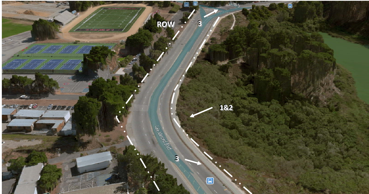
Figure B2 – Lake Merced Blvd looking from Middlefield to Winston
