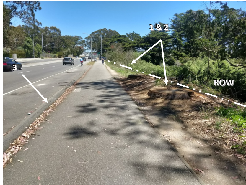
Figure H11 – Skyline Boulevard (SR 35) at end of bus pullout (ZOO Stop)
