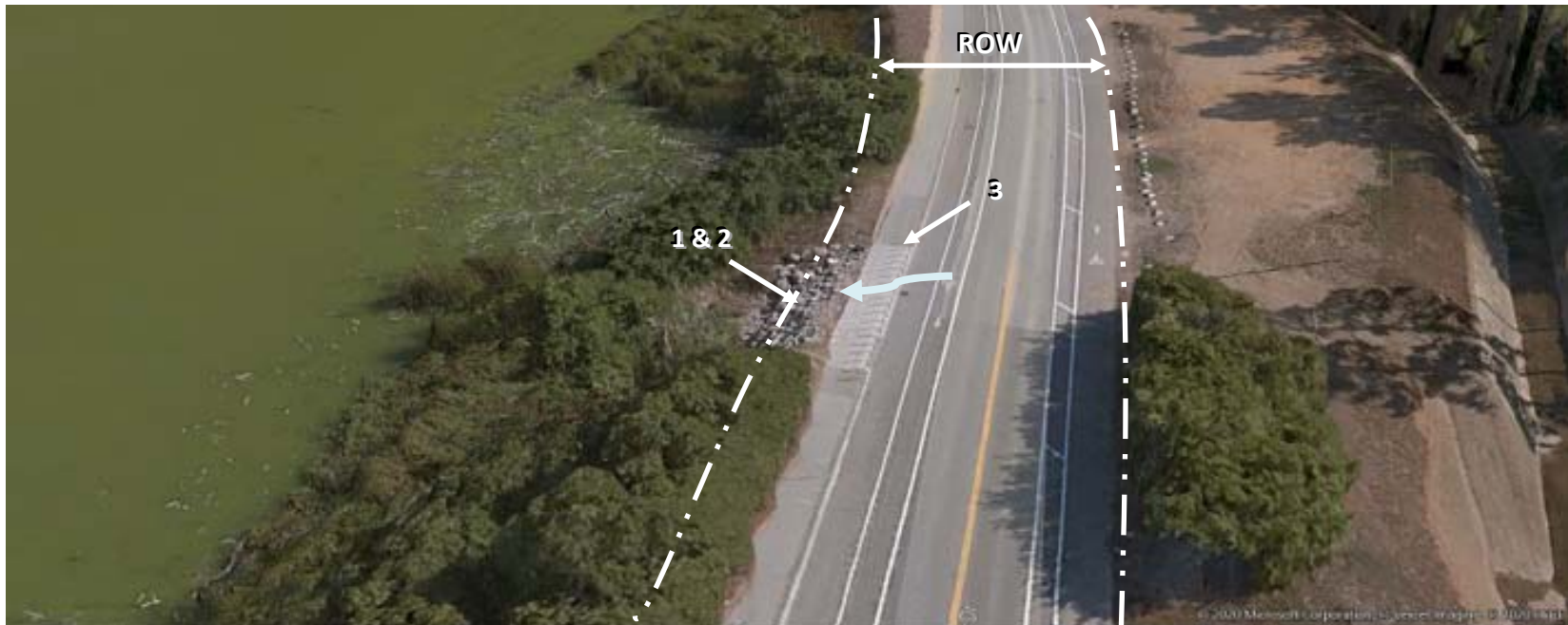
Figure F1 - John Muir Drive Erosion Control Structure No. 1 (Vista Grande Canal is visible to the right)
