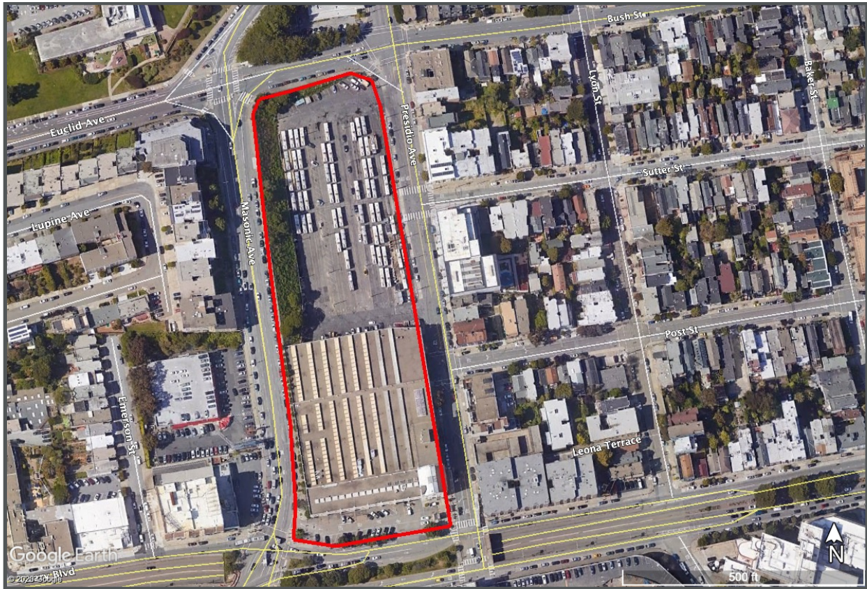
Figure 4-15. Presidio Yard - Existing Conditions (Aerial)
