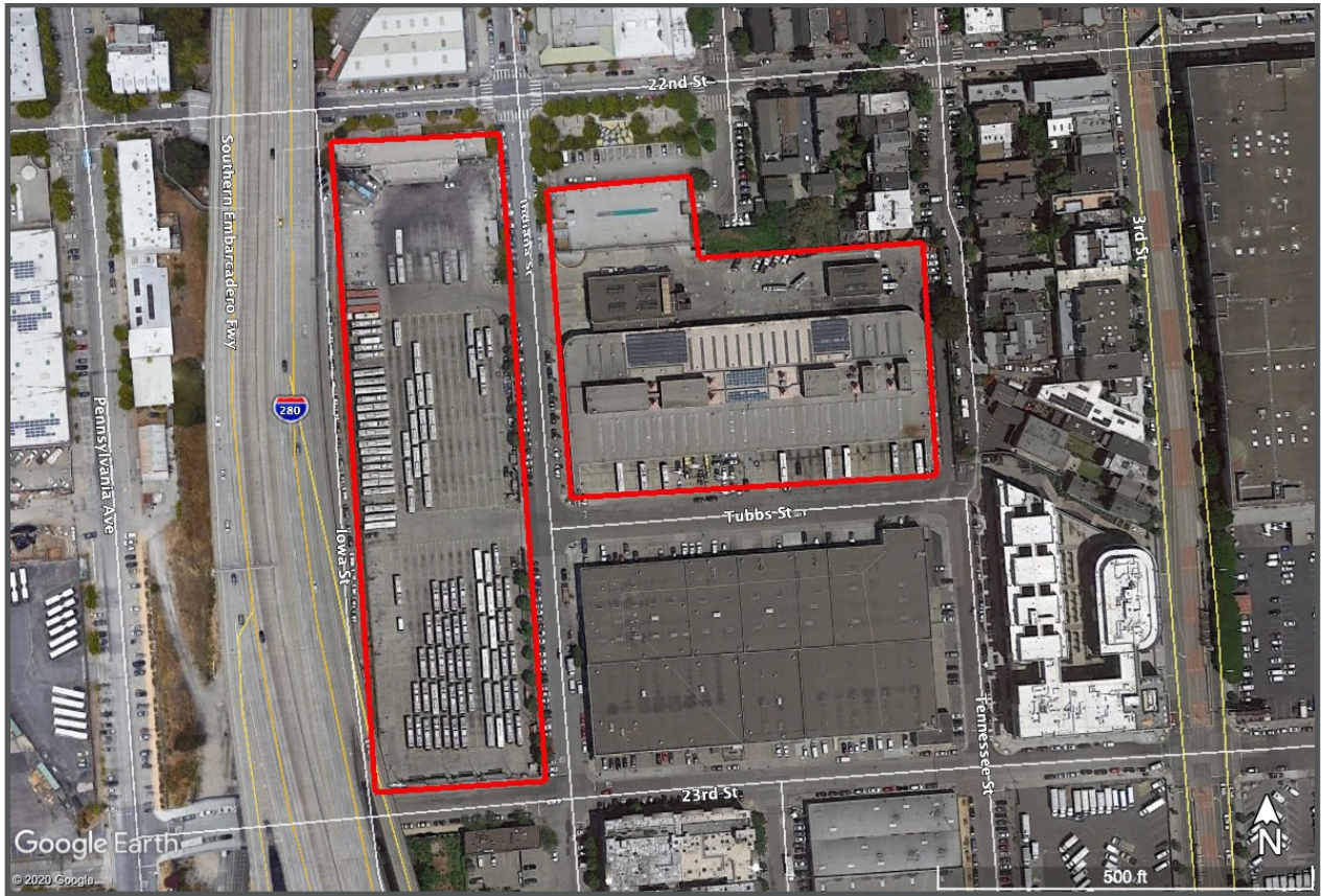
Figure 4-16. Woods Yard - Existing Conditions (Aerial)
