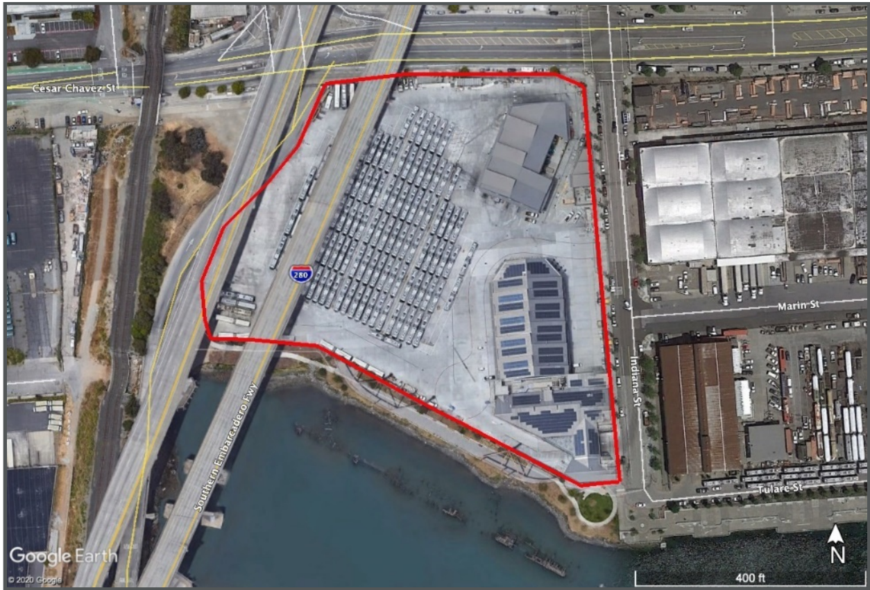
Figure 4-8. Islais Creek Yard - Existing Conditions (Aerial)
