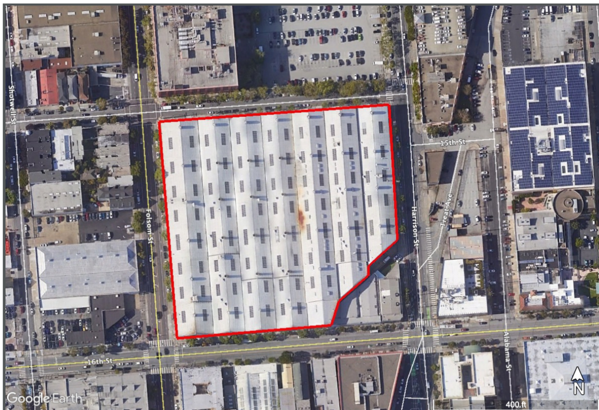
Figure 4-5. Flynn Yard - Existing Conditions (Aerial)
