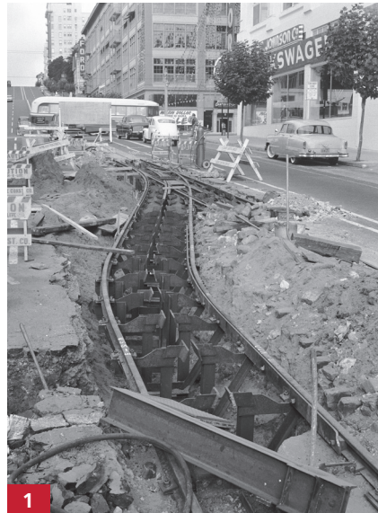
When the California Street Cable Car was reduced to its current length, a new turnout was built for it at California and Van Ness in 1957 (photo 1), and trial runs were taken at the end of the year (photo 2). Rails and Belgian Blocks used for street paving were recently uncovered during excavations for the Van Ness Improvement Project (photos 3 and 4).
