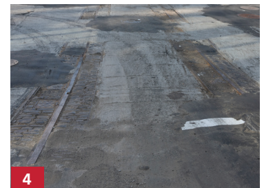
When the California Street Cable Car was reduced to its current length, a new turnout was built for it at California and Van Ness in 1957 (photo 1), and trial runs were taken at the end of the year (photo 2). Rails and Belgian Blocks used for street paving were recently uncovered during excavations for the Van Ness Improvement Project (photos 3 and 4).
