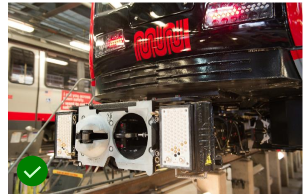
✓ Inspected and realigned over 130 Breda couplers
