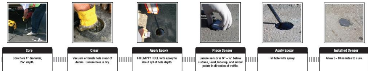
Roadway sensor installation process
