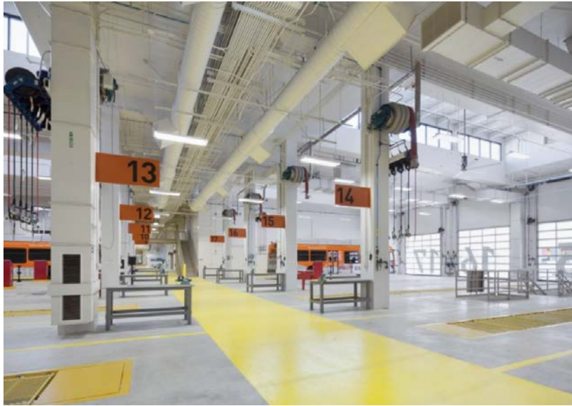
Drive-Thru Maintenance Bays
