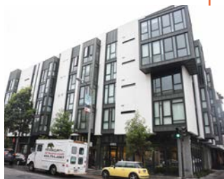
Adjacent building typology and character: five-story mixed-use modern development.
