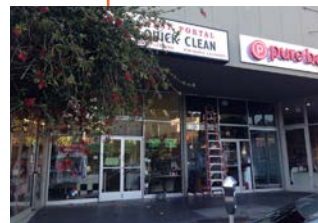
Adjacent storefront conditions.
