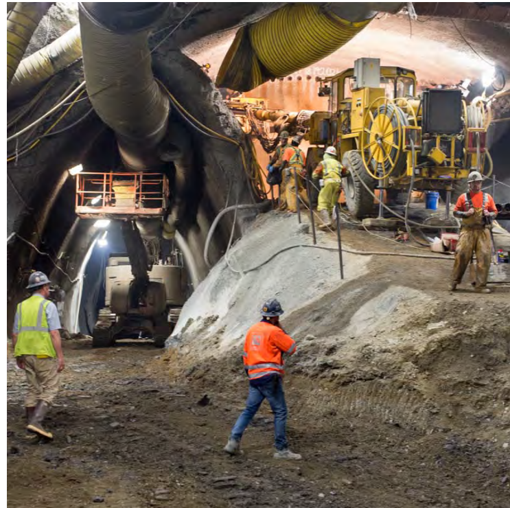
3 Excavation progresses one section at a time until it is finished
