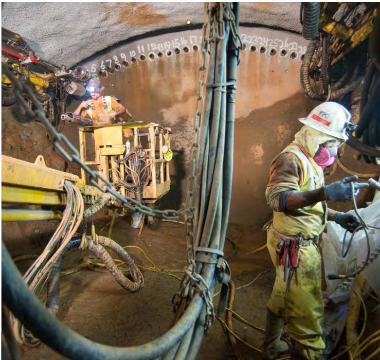
2 Drilling and soil improvement work are conducted for the ceiling arch
