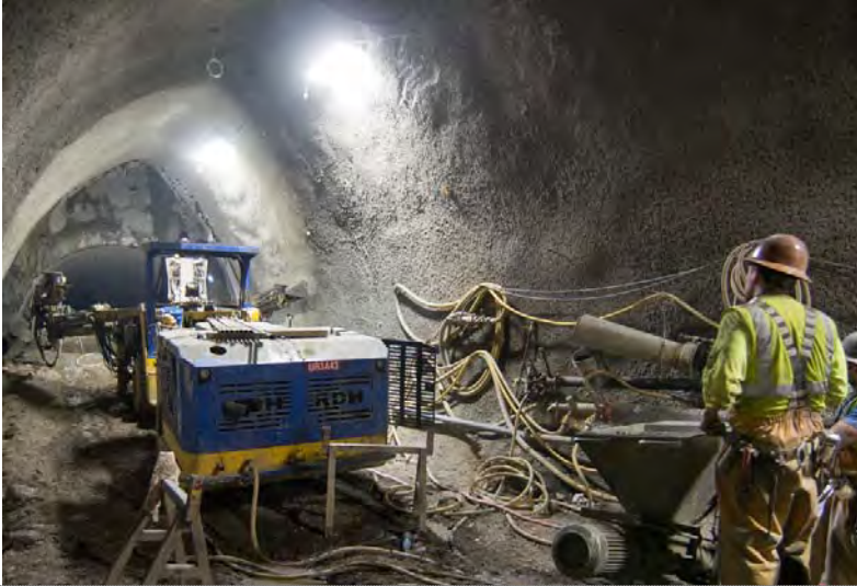
1 Side drifts are excavated
