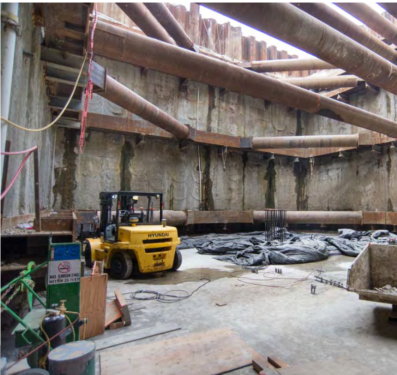
2 The slab is cleared, and work re-oriented to construct internal walls
