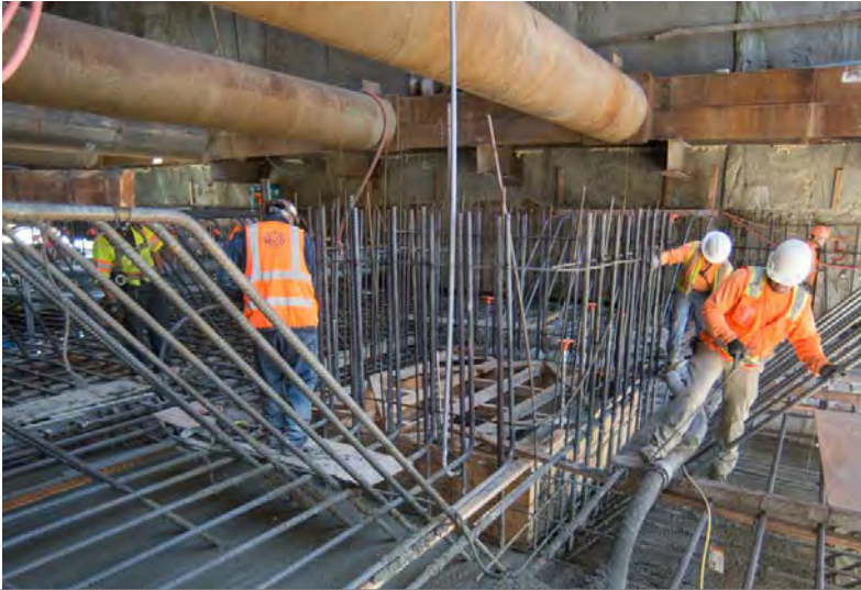
1 Final sections of rebar are installed, and concrete is poured
