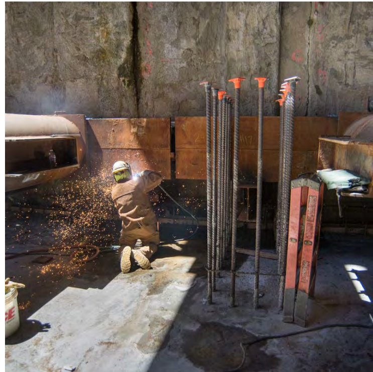
3 Workers begin removing temporary bracing on the lowest levels
