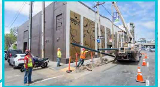
4th St. Surface Track, Systems (STS)
