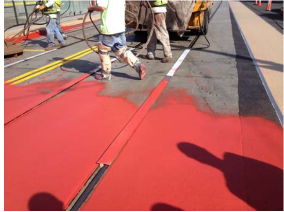
Application of Spray Coating
