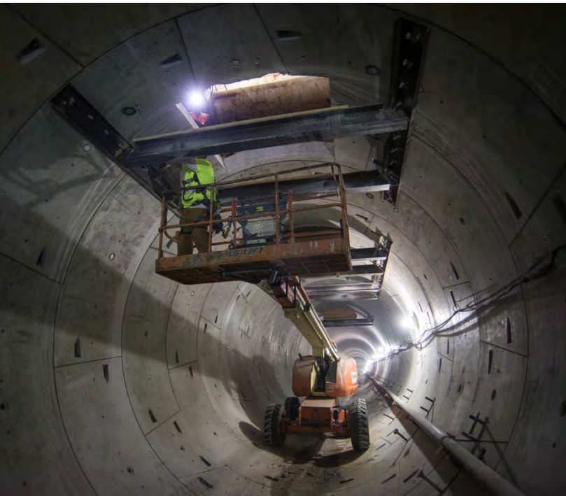
2 Steel bracing is installed in the tunnels to reinforce their structure
