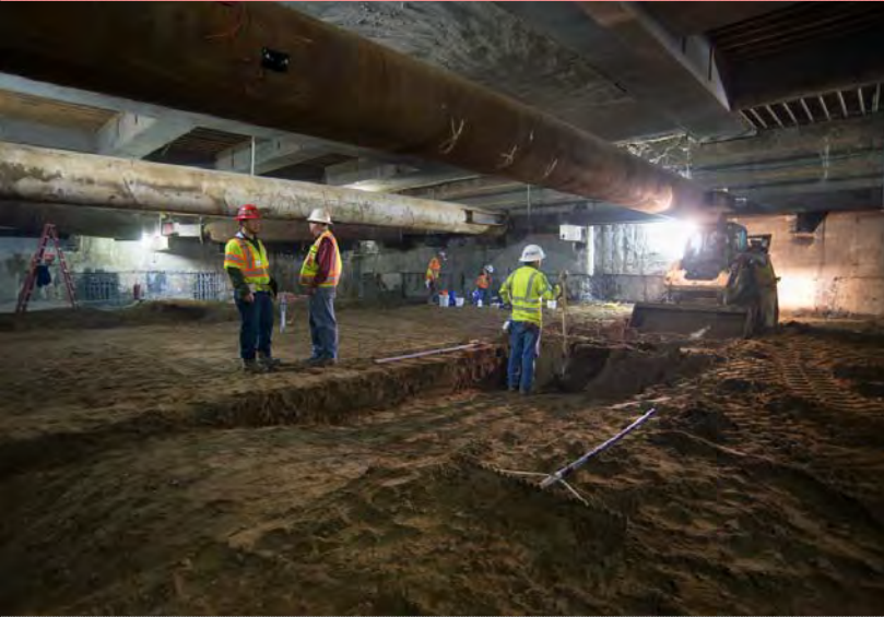
1 Workers carefully uncover the tunnels using small equipment
