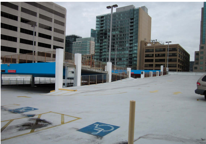
View on the Roof Level
