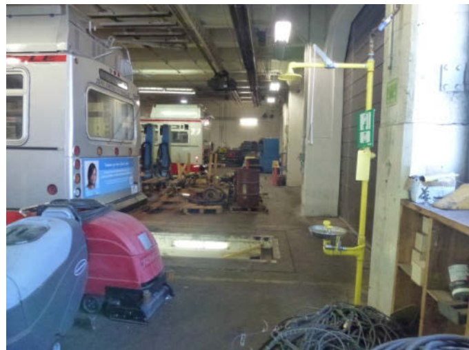
Forty Foot Bus Maintenance Area
