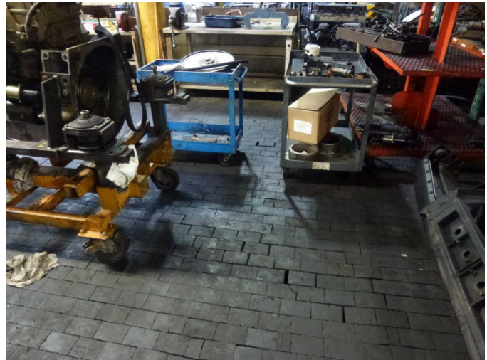
Machine Shop Wood Block Floors
