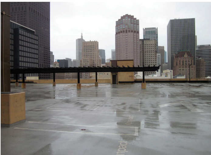
View on the Roof Level
