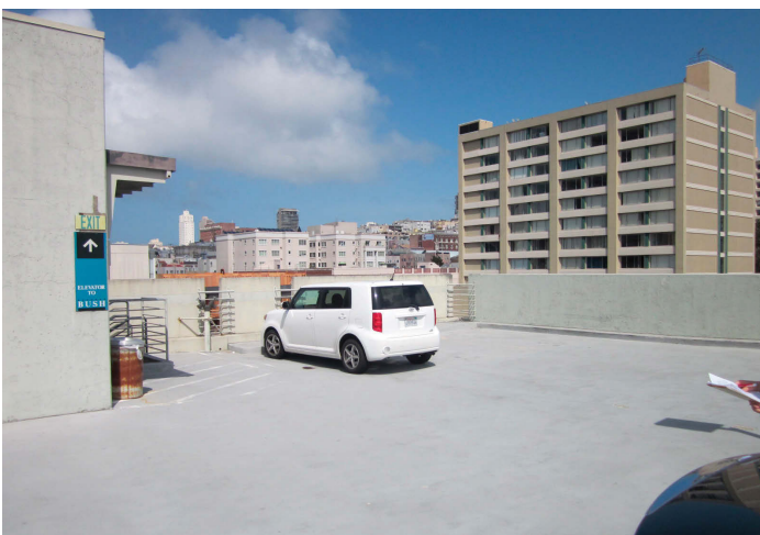
View on the Roof Level
