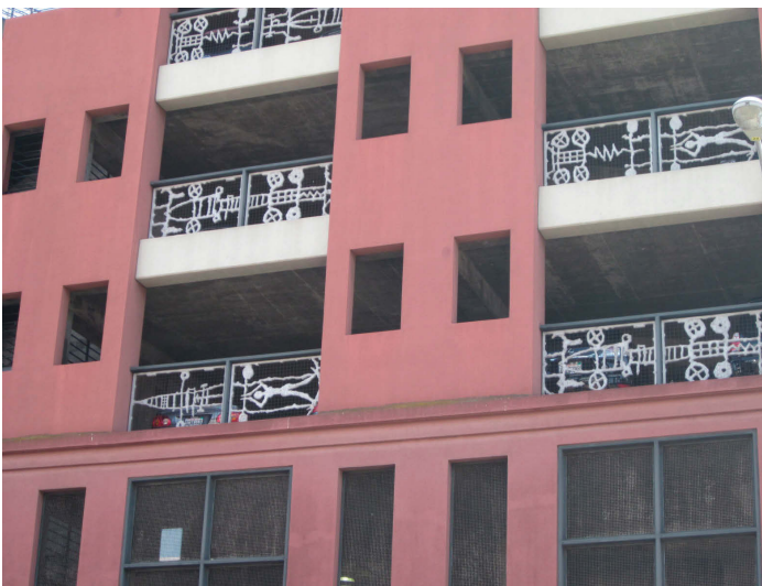
The Garage Facade
