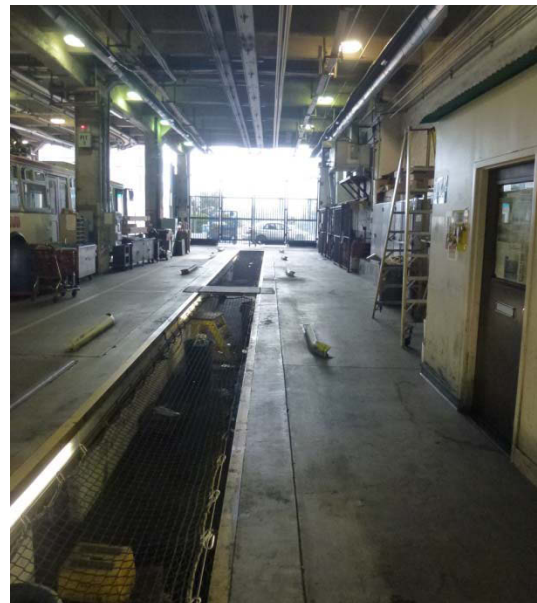
Repair Bay Pit
