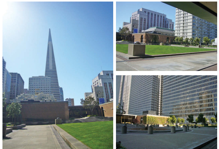
View on the Roof Level -Roof Plaza
