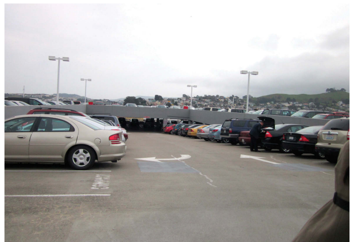
View on the Roof Level
