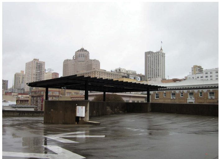
View on the Roof Level
