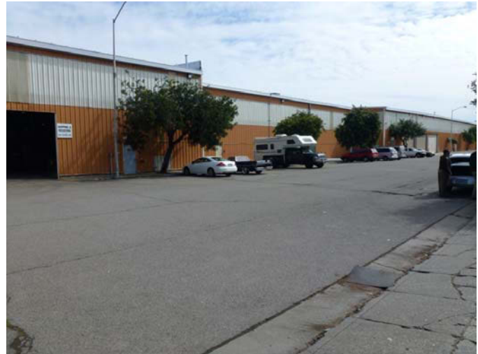
Burke Exterior and Employee Parking
