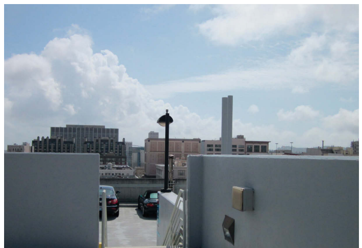
View on the Roof Level
