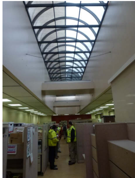
Administrative Offices - Skylight
