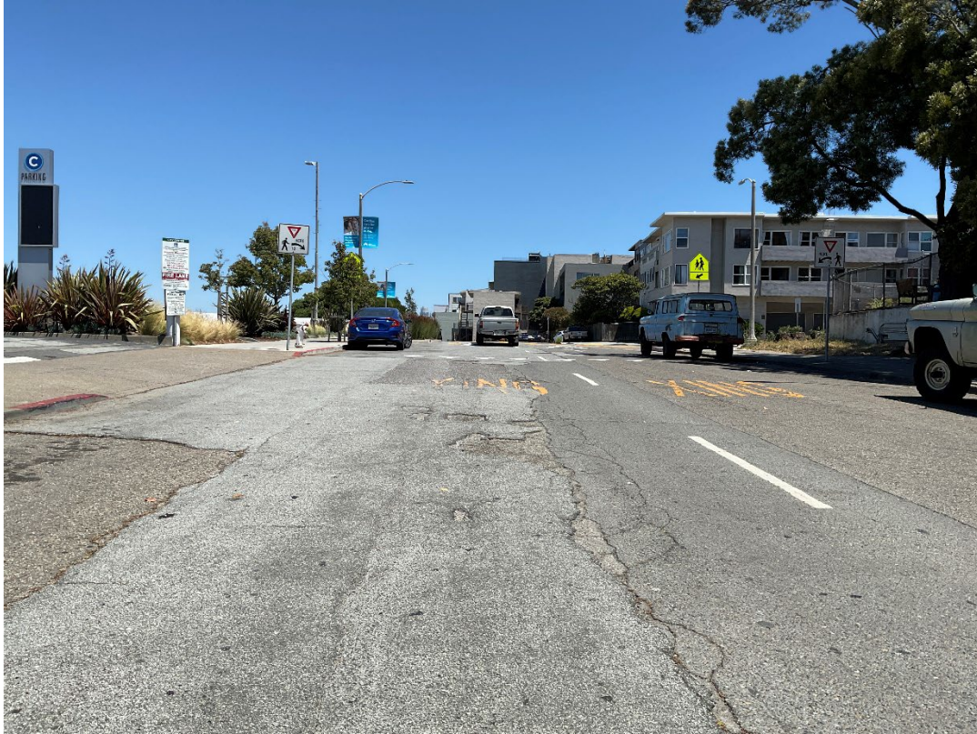
Figure 3: O'Farrell St at Anzavista Ave, eastbound, lane 1
