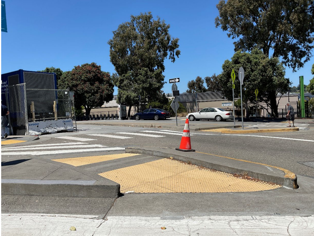
Figure 9: O'Farrell St at St Josephs St, eastbound looking left
