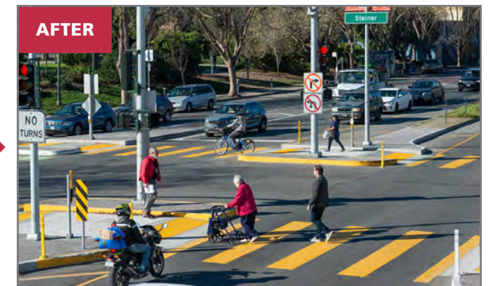
A better at-grade crossing at Steiner Street (after): The pedestrian bridge (left) was replaced with accessible, clearly marked at-grade crossings along both sides of Geary Boulevard, including pedestrian refuge islands.
