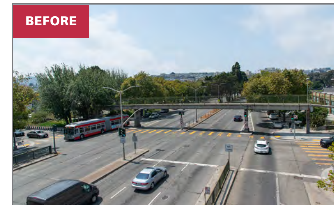
Pedestrian bridge at Steiner Street (before): This pedestrian bridge, which was not compliant with the Americans with Disabilities Act, made it difficult to cross Geary Boulevard. Only one side of Geary Boulevard had a street-level crosswalk.
