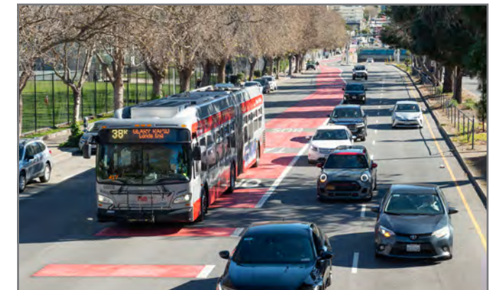
Red transit lane on Geary Boulevard: Red transit lanes were installed in the Western Addition as part of the Geary Rapid Project.
