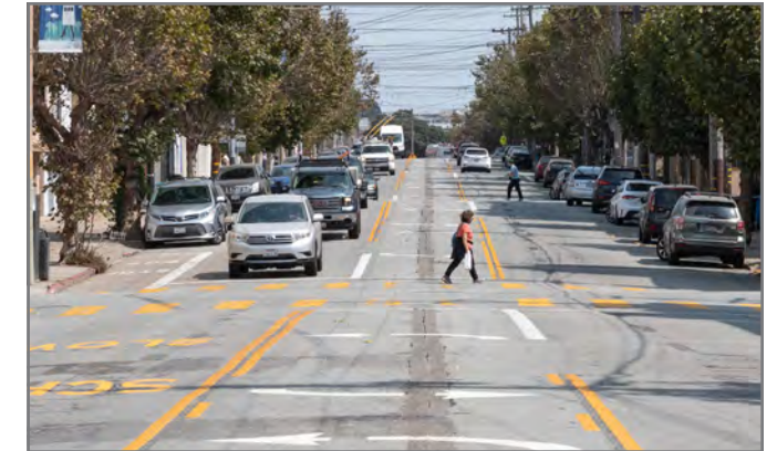
California Street "road diet" in the Inner Richmond: Muni Forward removed a general purpose lane to better accommodate transit vehicles and calm traffic on a high-injury corridor.
