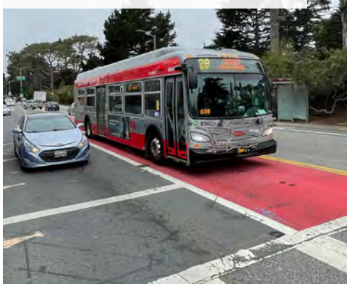
The 29 Sunset uses a transit queue jump on Lincoln Way at 19th Avenue.
