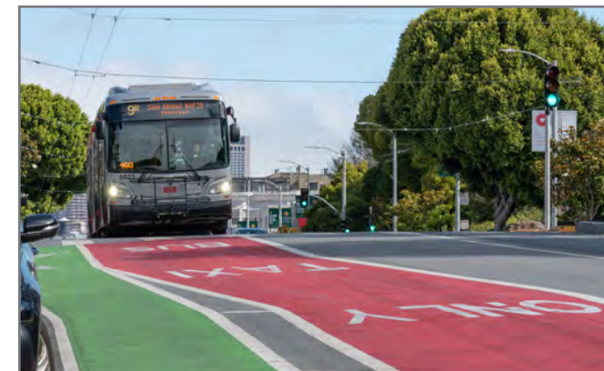
Red bus lane on Potrero Avenue: New red transit lanes and an upgraded bike lane were installed as part of the Potrero Avenue Streetscape Improvement Project.
