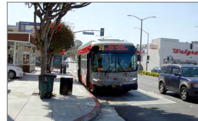
Bus bulbs on Lombard Street: These wider boarding platforms improve the rider experience and reduce delays on the 28 19th Avenue and 28R 19th Avenue Rapid.
