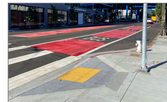
Pedestrian bulbs on 16th Street: Wider sidewalks at intersections shorten crossing distances and improve visibility, making intersections safer.
