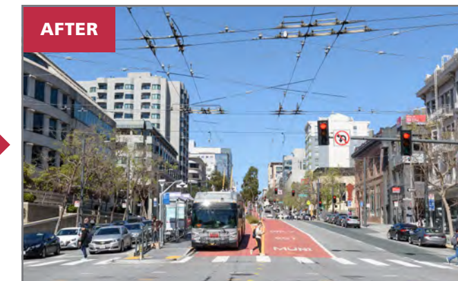
Van Ness Avenue at McAllister Street after Van Ness BRT opening (2022): The project features extensive safety features, including wider sidewalks at intersections and left turn restrictions.
