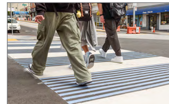
Decorative high-visibility crosswalk: Upgraded crosswalks on Taraval Street both improve safety and contribute to the unique streetscape, complementing Taraval's oceanside location.
