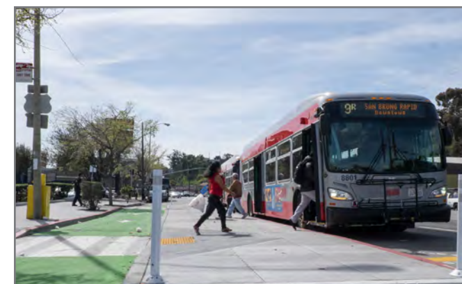
Transit island on Bayshore Boulevard at Flower Street: New transit islands adjacent to bike lanes along the 9R San Bruno Rapid route safely separate bikes from loading buses.
