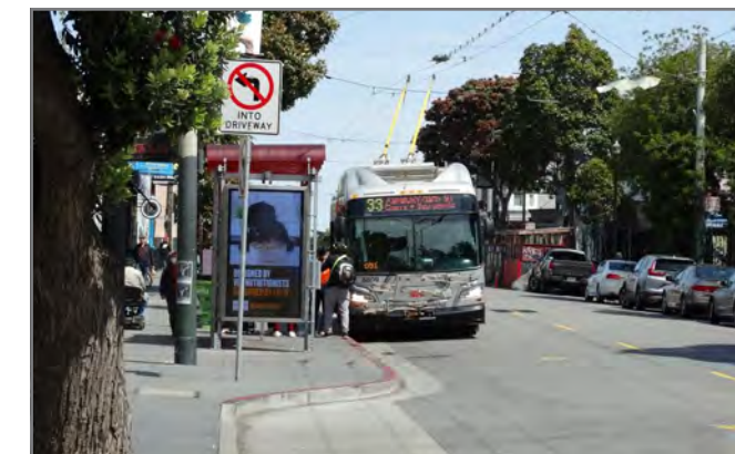
Wide boarding platforms on Haight Street: Transit bulbs on Haight Street, shown here at Stanyan Street, reduce boarding delays, improve safety and leave more space for stop amenities.
