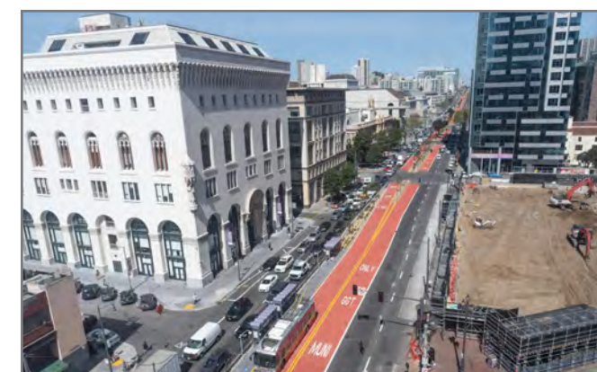
Van Ness BRT corridor, looking north from Market Street: The 49 Van Ness/Mission runs in center-running transit lanes for the length of Van Ness Avenue, eliminating most potential delays.
