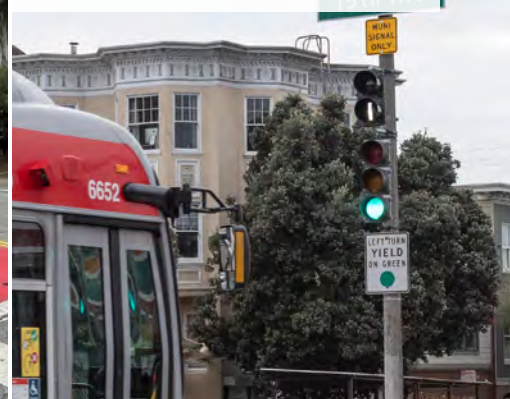
A transit queue jump traffic signal on Geary Boulevard.
