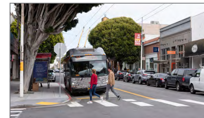
Bus bulb in Marina District: Bus bulbs were installed at stops on Chestnut Street to help riders get on and off the bus more quickly, easily and safely.
