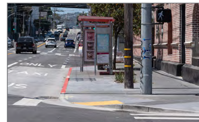
Transit bulbs on 16th Street: Wider boarding platforms on 16th Street provide a better waiting environment for riders and help to reduce delay.
