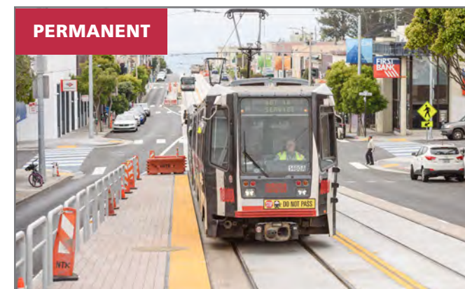
Permanent transit boarding islands on Taraval: Quick-build safety zones have been replaced with new permanent boarding islands made of concrete at all stops on Taraval Street.
