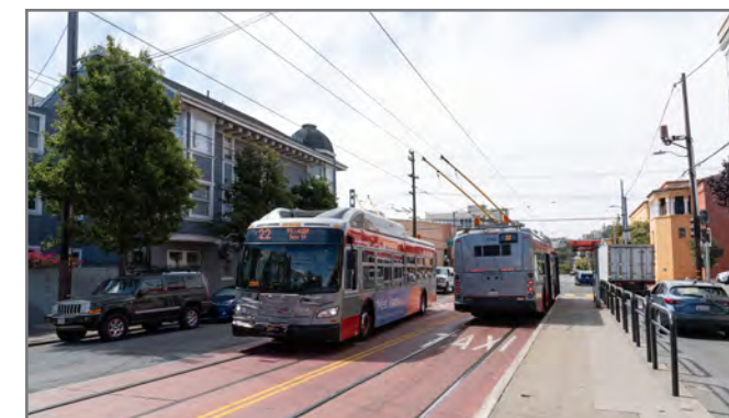
Church Street red transit lane: Total travel time on Church Street dropped by up to 14% or one minute (median) and travel time variability dropped by up to 27%. (Source: Church Street Pilot Transit Lanes , 2015, SFMTA)
