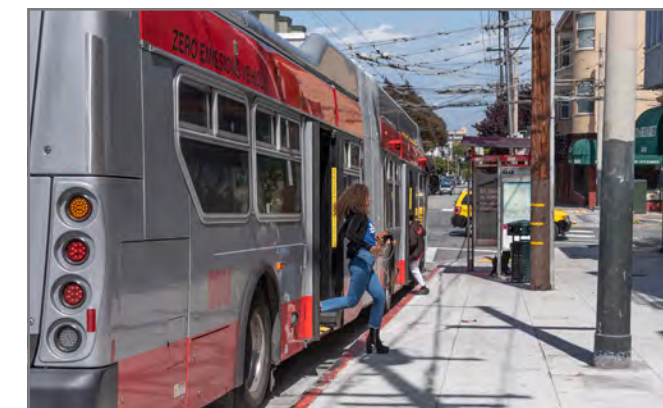
Permanent concrete transit bulbs on Fulton and McAllister streets: New transit bulbs—shown here at McAllister and Divisadero streets—help to improve travel time and safety.
