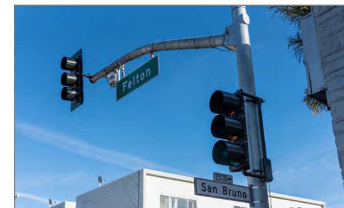
New traffic signal on San Bruno Avenue: A new traffic signal with transit signal priority replaced a stop sign at San Bruno Avenue and Felton Street.
