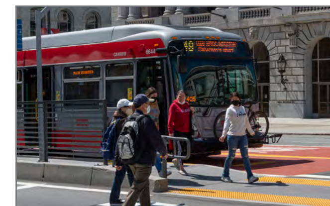
Center boarding island platforms: Passengers get on and off the bus by walking to a transit island. These boarding islands enable the bus to operate in center-running transit lanes.
