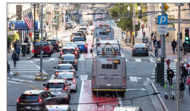
Stockton Street red transit lane: An existing transit lane on Stockton Street in Union Square was upgraded with red colorization to improve driver compliance in this busy corridor.
