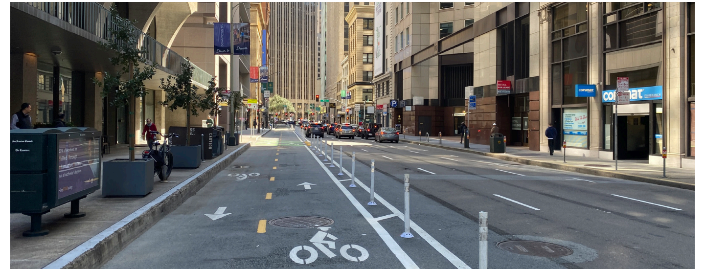
After Quick-Build Improvements on Battery Street
