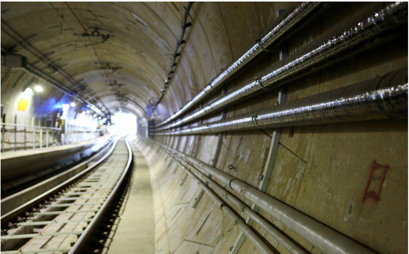
View of STS Portal
