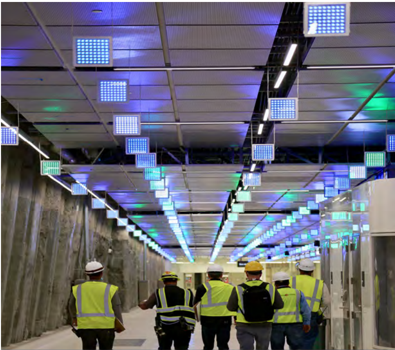
Platform entrance from Concourse escalators
