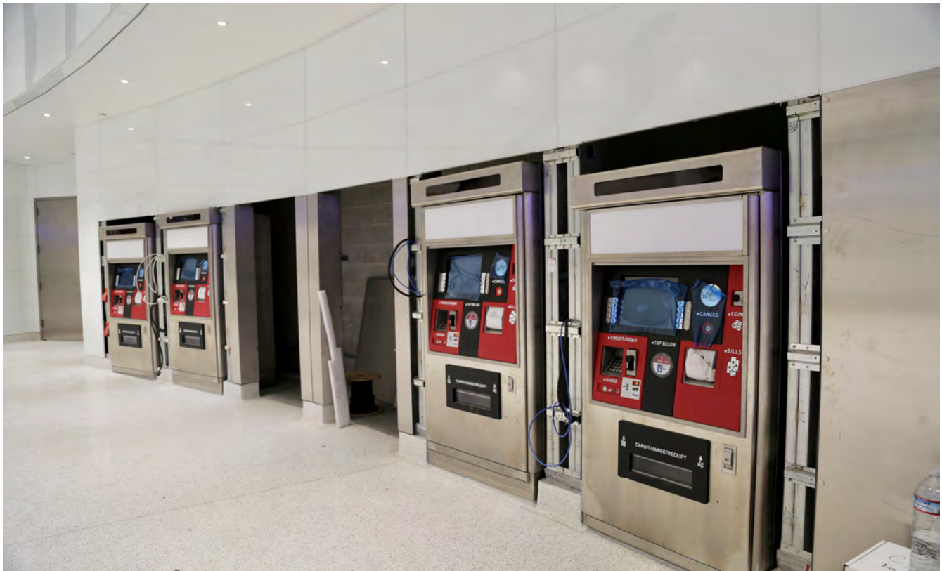
UMS Concourse Level ticket booth installation
