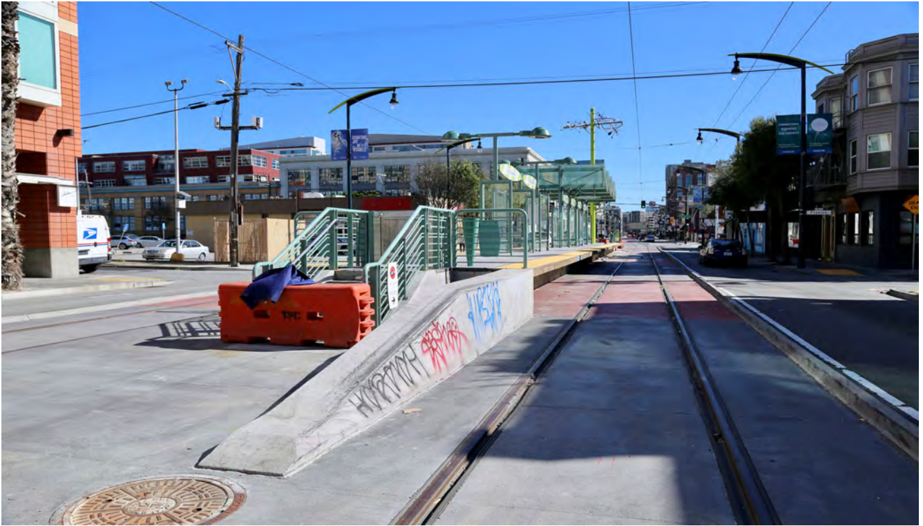
STS Platform on 4th Street
