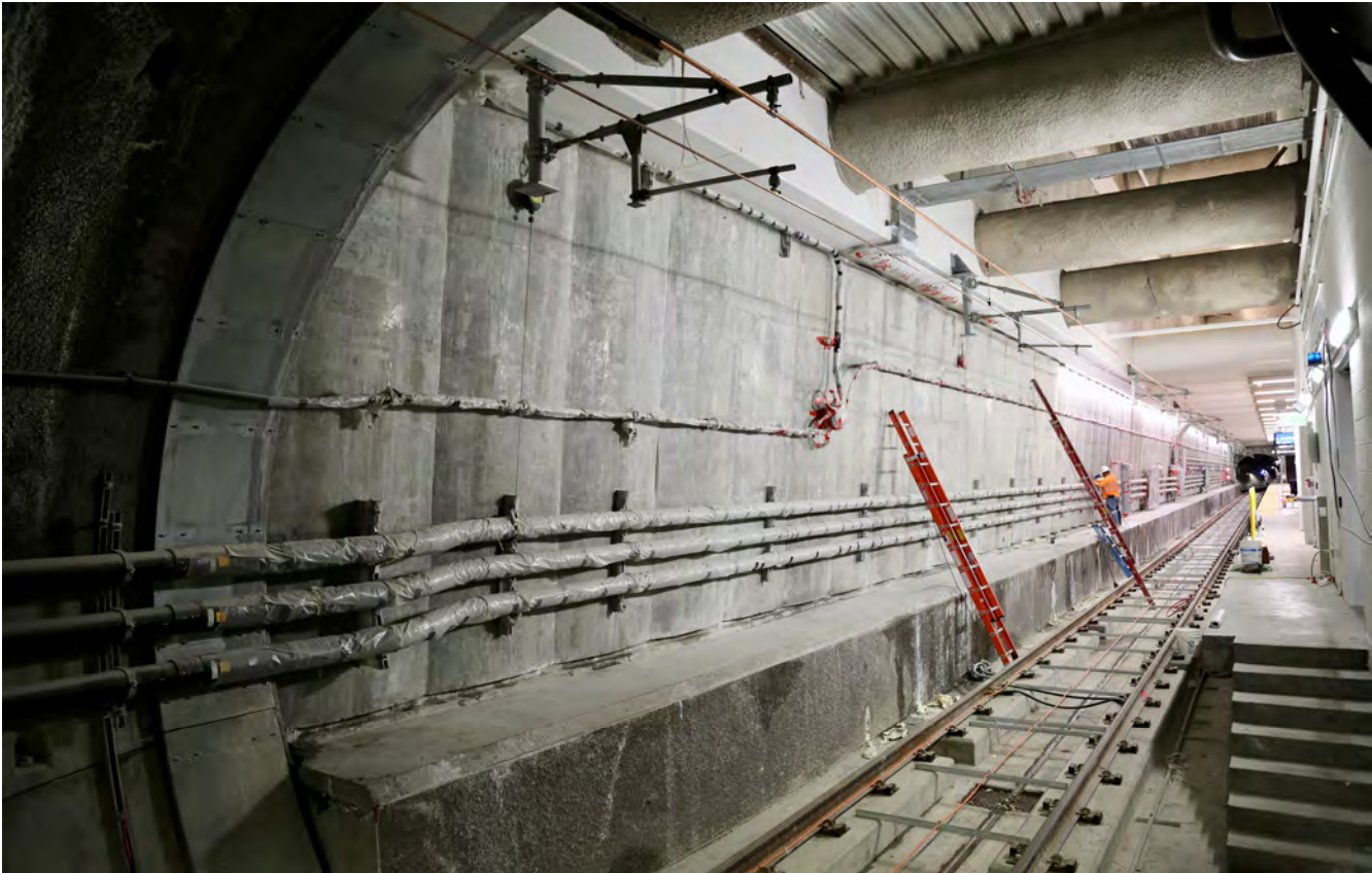
UMS view of Northbound Tunnel looking South
