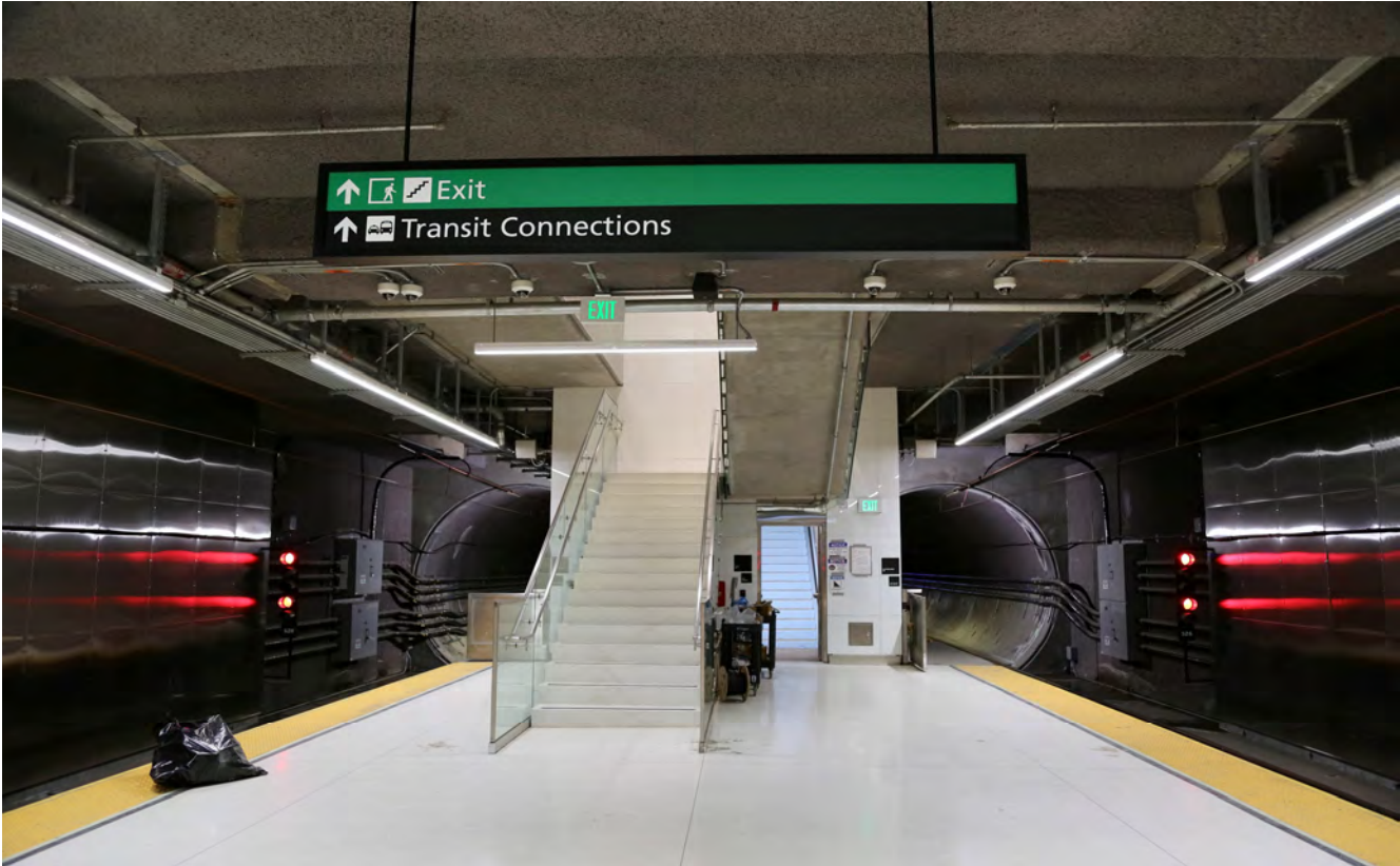
Stairs to Platform Level with installed traffic lights
