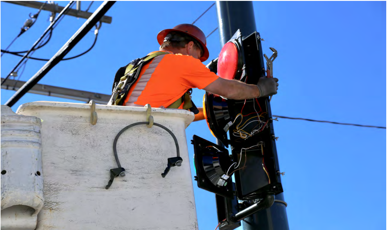
Surface traffic signal installation
