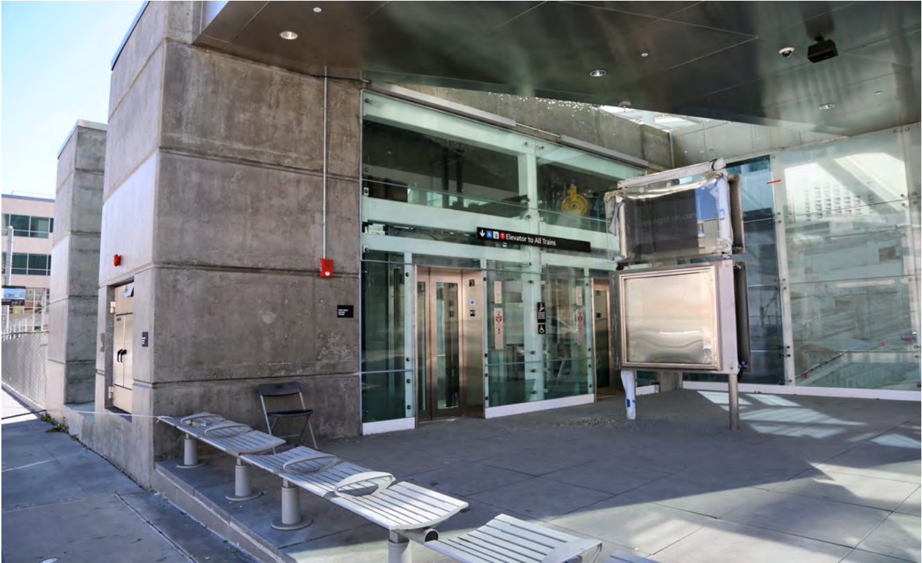
Surface level elevators and glass art
