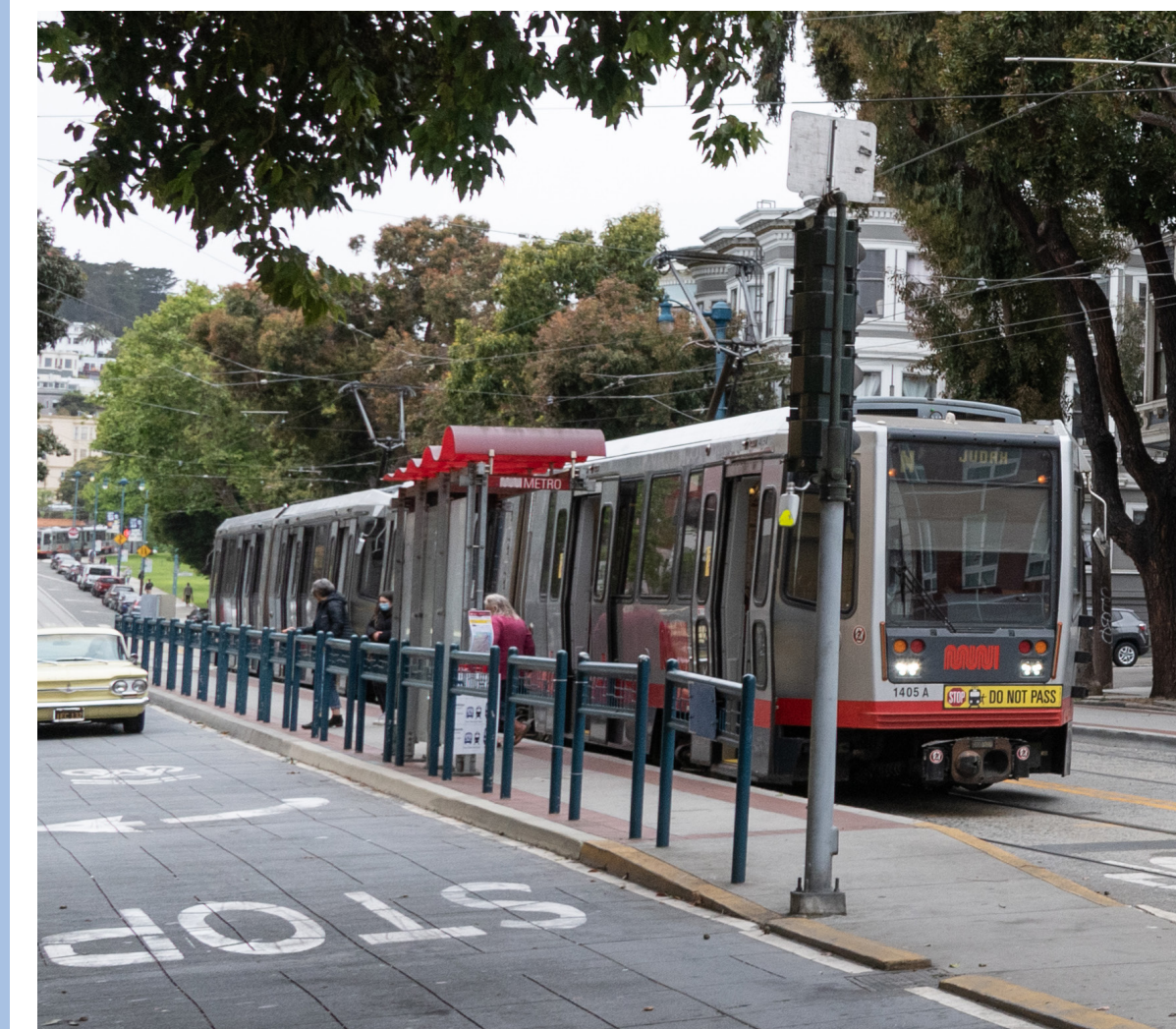
Extend and upgrade platforms
