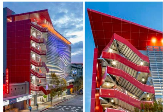
Figure 7. Expressed stair and perforated metal facade provides visual interest. Example: Center Street Parking Garage, Berkeley, CA.
