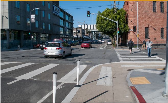
Paint, signs, and delineators
