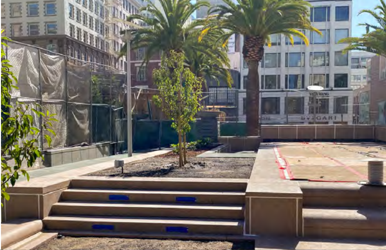
Waterproofing, terrace blocks, and landscaping are completed.
