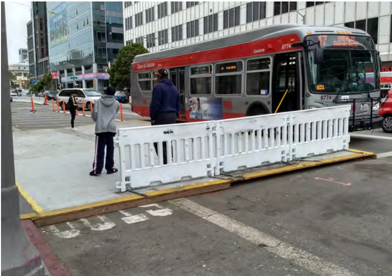
Temporary bus bulbs
