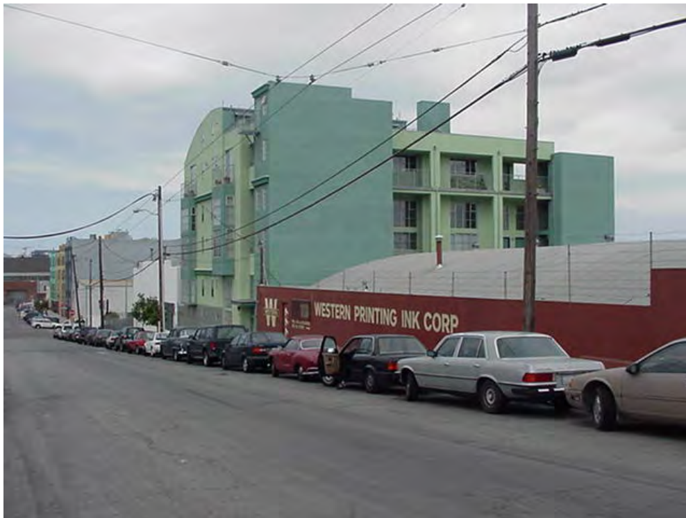
Photograph No. 8: Tennessee Street between Nineteenth Street and Eighteenth Street
