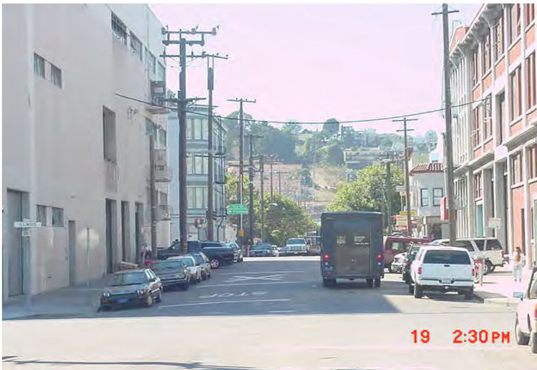
Photograph No. 24: Twenty-Second Street between Illinois Street and Third Street
