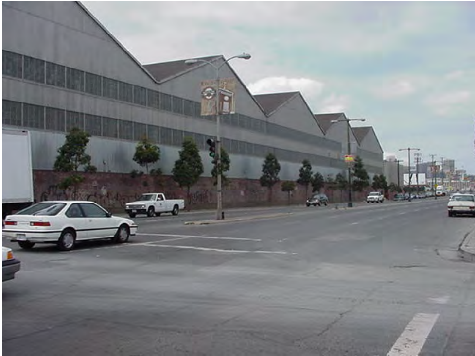
Photograph No. 1: Intersection of Third Street and Mariposa Street
