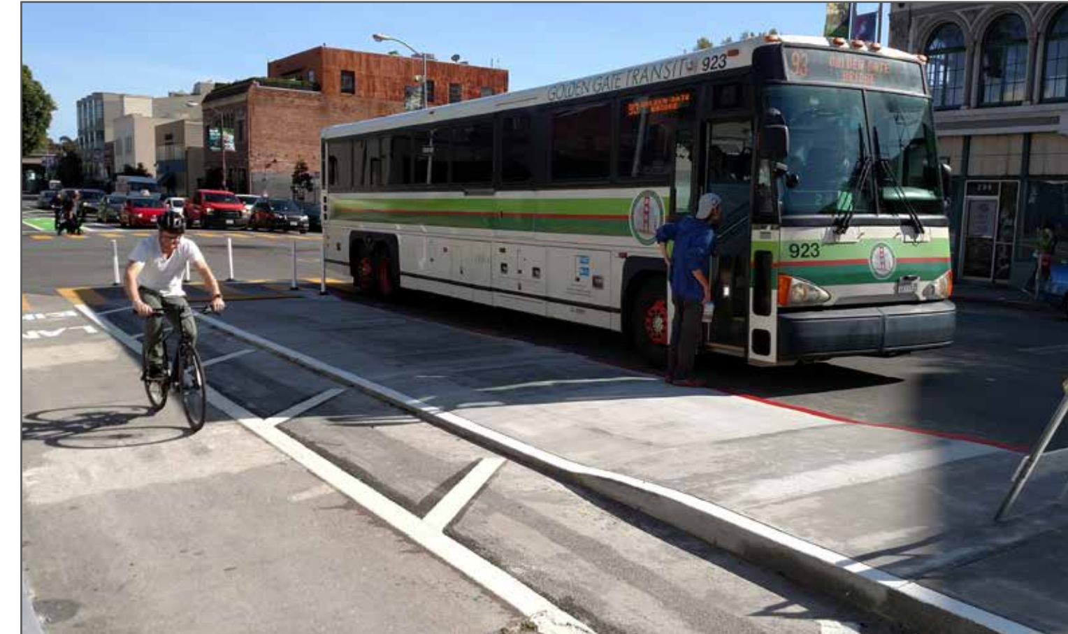
Boarding islands will reduce conflicts between the 12-Folsom and bicycle riders while decreasing travel time and improving reliability.
