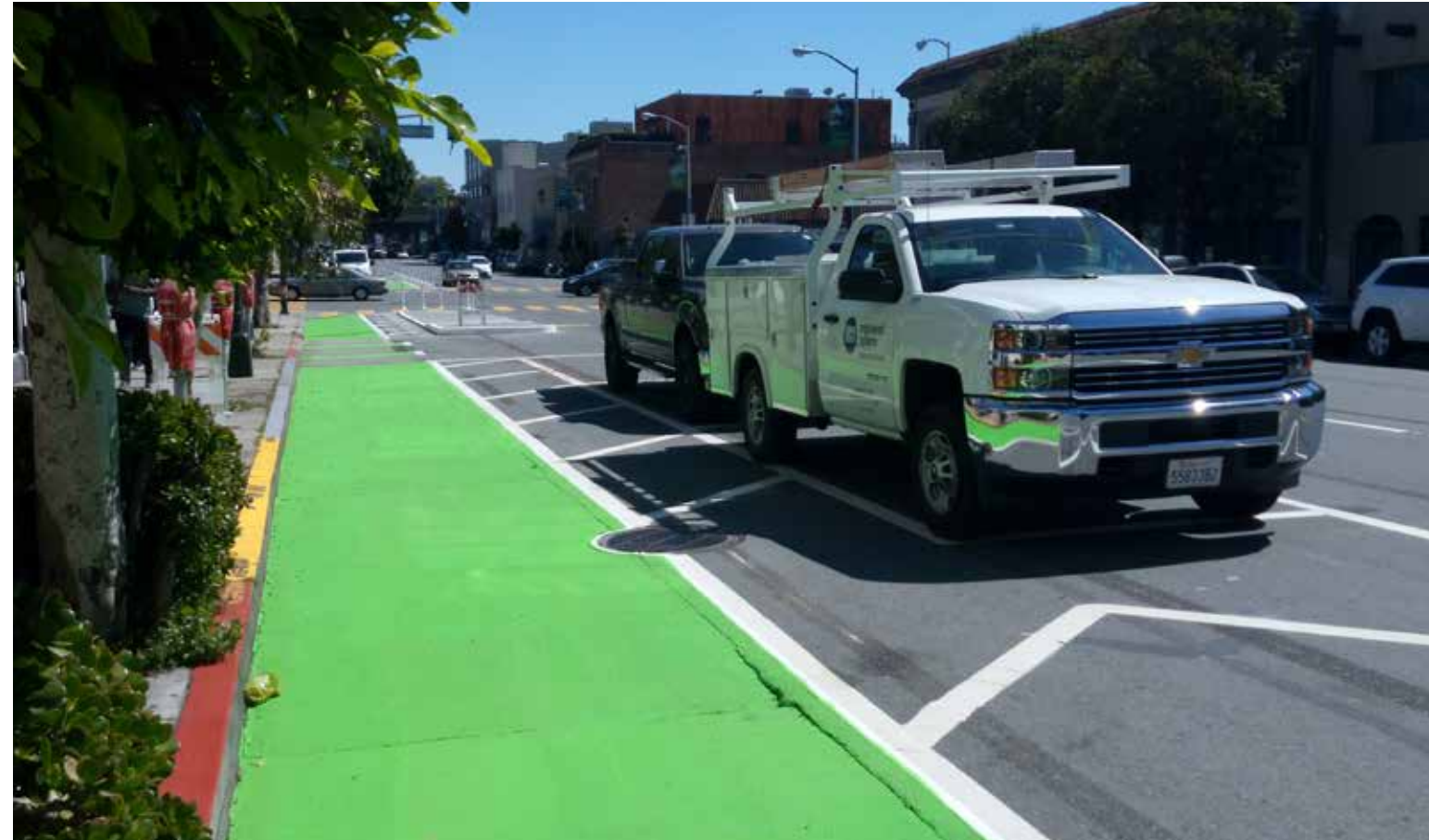
Parking protected bikeways separate pedestrians and bicyclists from cars. They also reduce vehicles blocking bike lanes - currently, a frequent problem.
