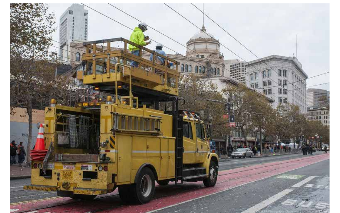
Overhead wire maintenance
