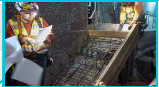
4th St. Surface Track, Systems (STS)
