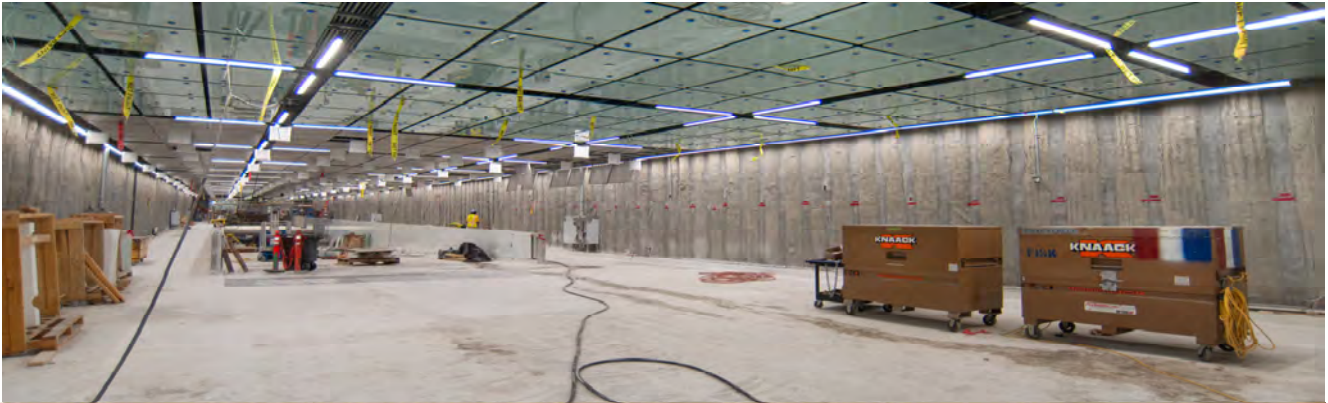
Lighting and glass ceiling panels have been installed inside the south concourse for Union Square/Market Street Station.
