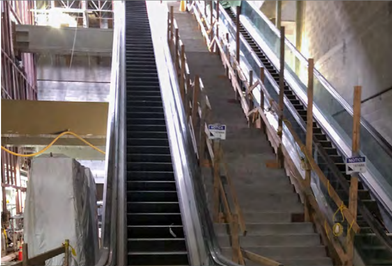
All escalators have now been placed inside Rose Pak-Chinatown Station.
