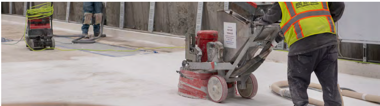
Two men work to smooth a section of terrazzo floor inside the center concourse for Union Square/ Market Street Station.
