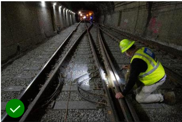
Conducted critical inspections and maintenance
