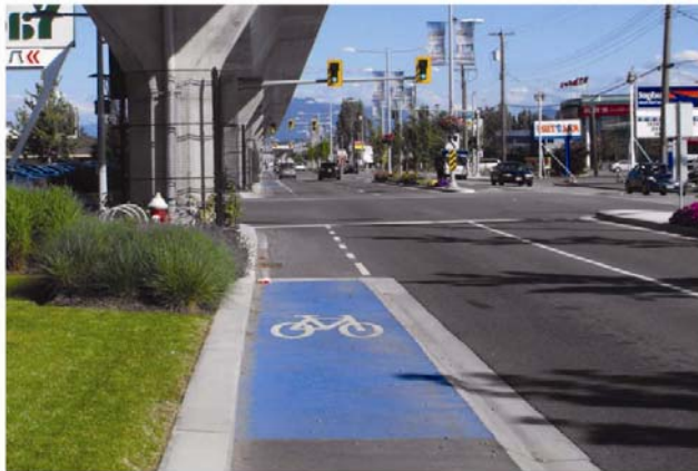
Cycle track next to traffic lanes (Vancouver, BC)
