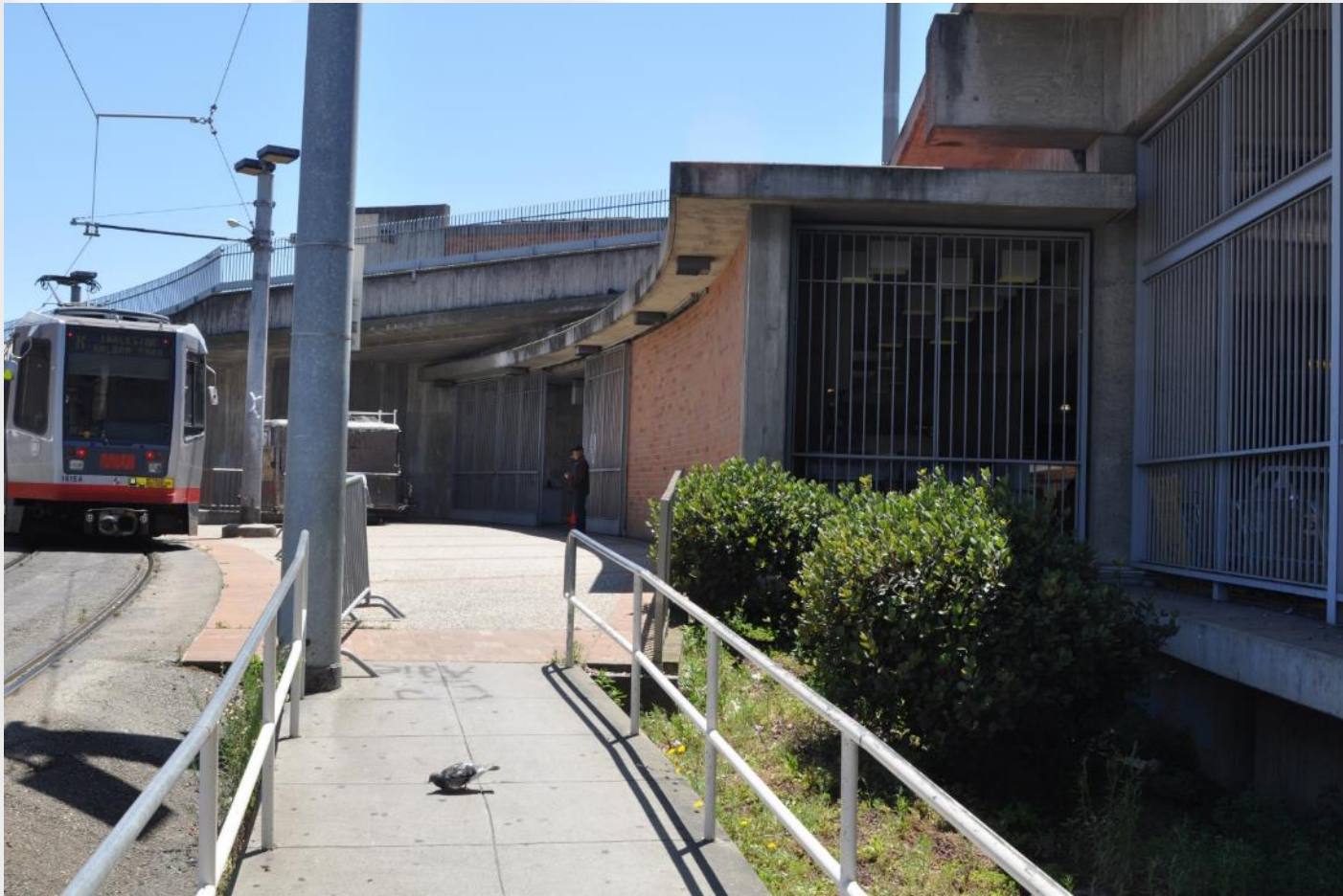
Concourse walkway to South Entry (free area) – Existing Condition
