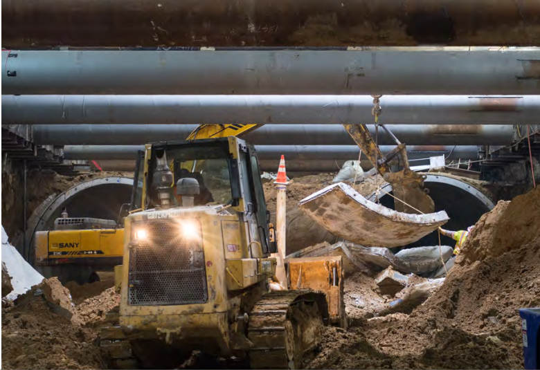
1 Crews excavate and remove tunnel segments from the platform level
