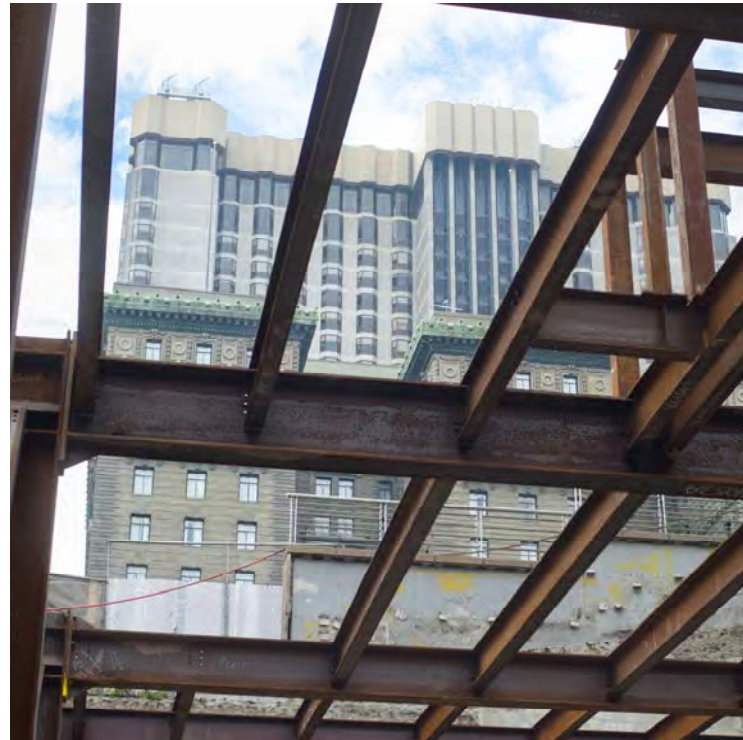
3 Steel members are installed
