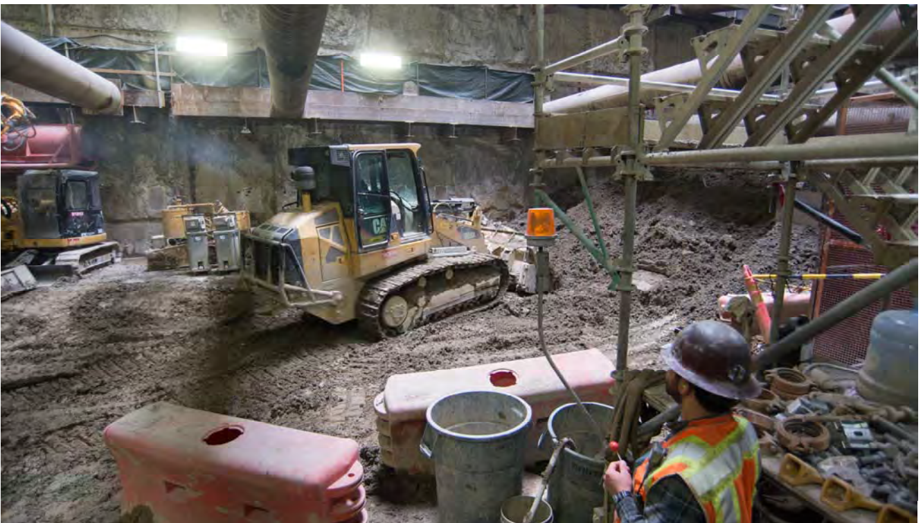
A bulldozer operator collects material to be lifted to the surface, under the main access shaft of the station headhouse.
