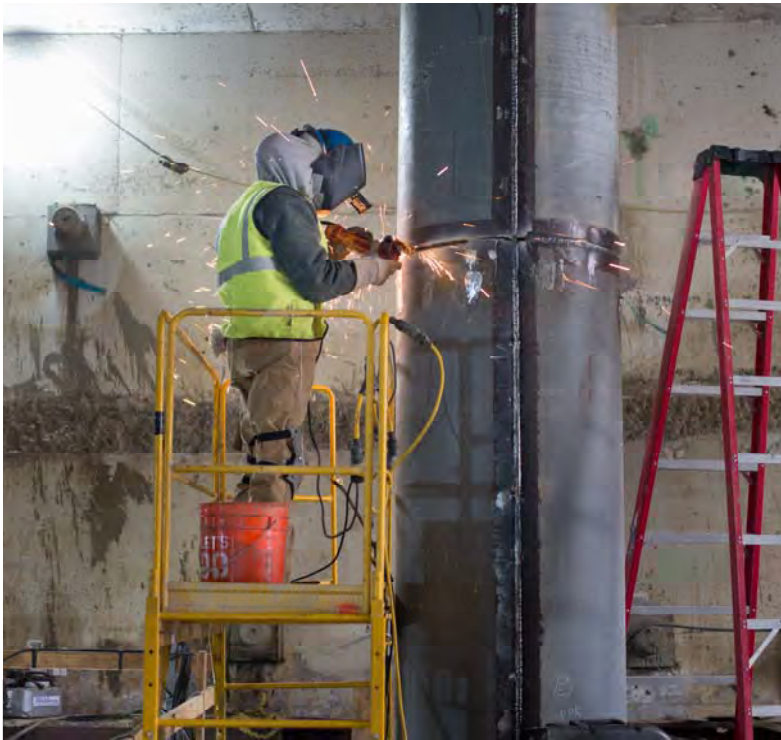
2 Existing columns and structural elements are reinforced
