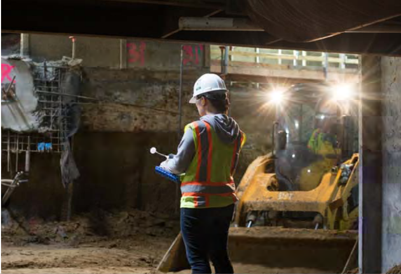
1 The site is graded and a concrete slab is poured
