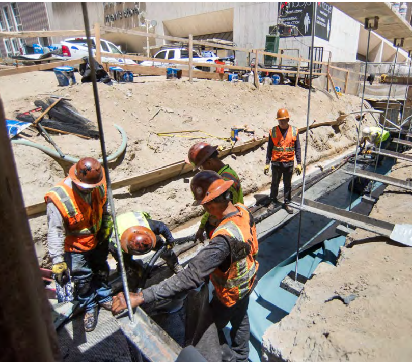
2 Concrete is poured and waterproofing is installed
