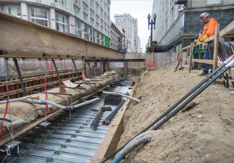
1 Workers install corrugated steel panels below utilities suspended above
