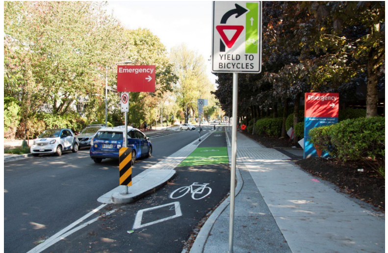
Figure 7: Protected Bike Lane in Vancouver, BC outside an Emergency Room provides horizontal and vertical deflection at the conflict point.
