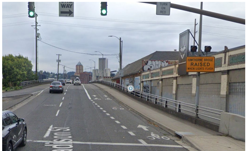
Figure 3: Example of a passing lane on a high-volume inclined bike lane
