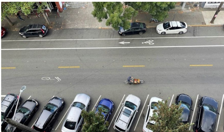
Figure 9: Example of an uphill climbing lane with shared lane markings in the downhill direction
