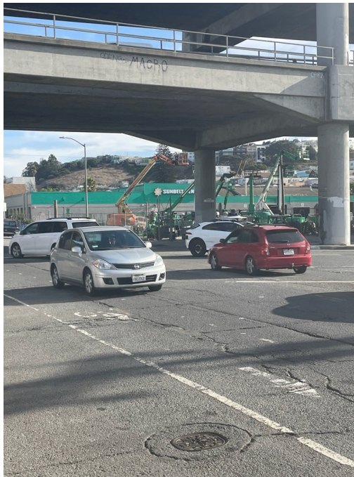
Intersection of Oakdale/Industrial (Unsafe Bike Lanes)
