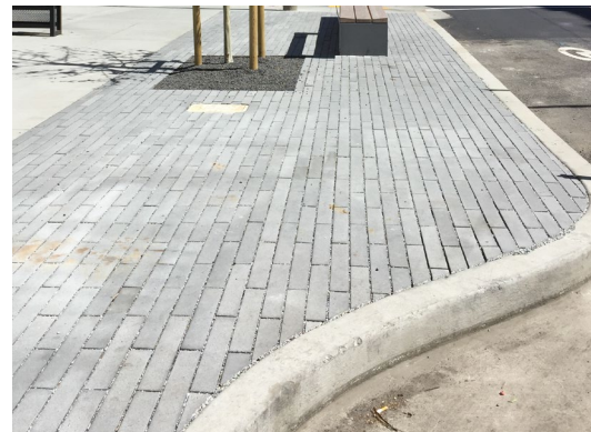
CORNER CURB BULB OUT
