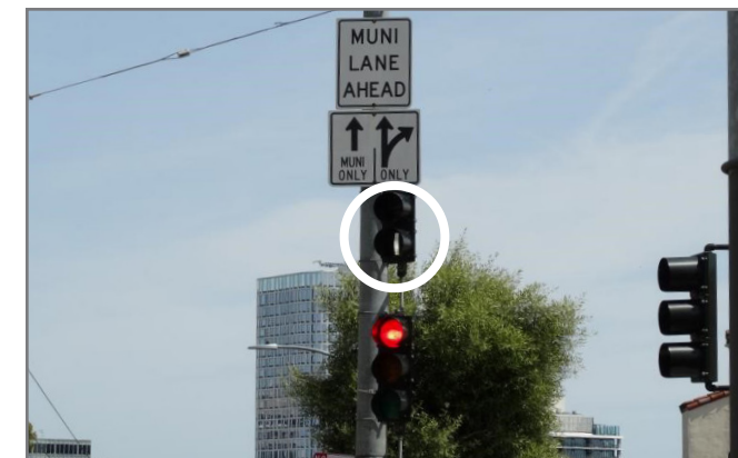
Head start for buses on Haight Street at Buchanan Street: This "queue jump" signal helps buses transition into a center bus lane from the curb. The vertical white bar (circled) is a special signal for buses, which get a head start to enter the intersection.
