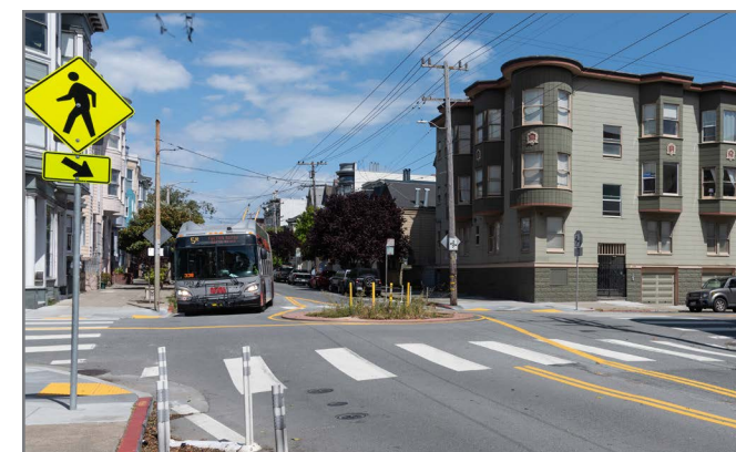
New transit-friendly traffic circle: A traffic circle replaced a four-way stop sign at McAllister and Lyon streets. Cross traffic must still stop and buses, traffic and bikes on McAllister have right-of-way.
