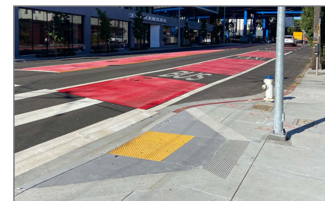
Pedestrian bulbs on 16th Street: Wider sidewalks at intersections shorten crossing distances and improve visibility, making intersections safer.
