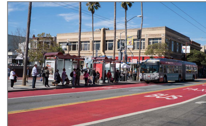
Red transit lane on Mission Street: A new red transit lane was installed in the Mission (shown at 24th Street) in 2016 to reduce delay, in tandem with other safety and reliability features.
