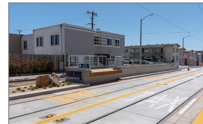
New wheelchair accessible boarding platforms and transit lanes on Taraval: These features have improved safety, accessibility and transit reliability on the L Taraval.
