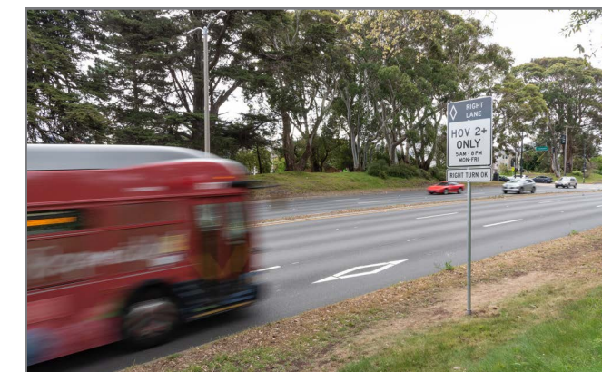
Park Presidio Boulevard HOV lane: The HOV lane pilot project on Park Presidio Boulevard provides benefits to both transit and people carpooling.
