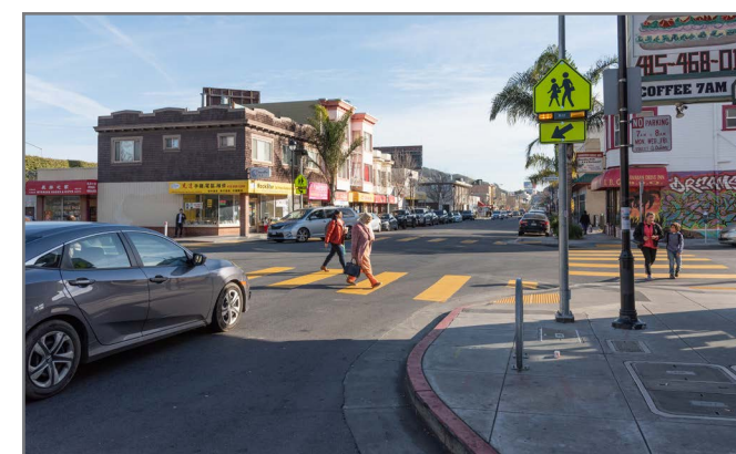
Pedestrian bulb on San Bruno Avenue at Burrows Street: New pedestrian bulbs and flashing beacons were installed as part of the San Bruno Avenue Multimodal Improvement Project.
