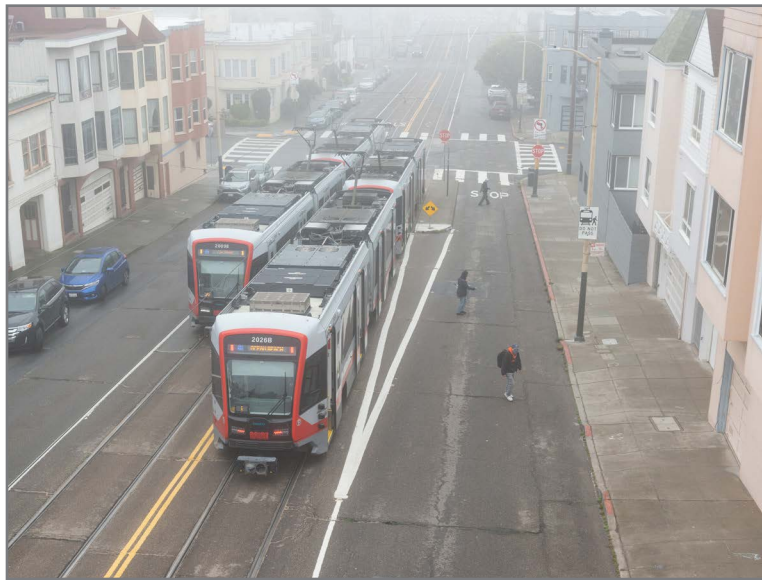
N Judah transit stop on Judah Street at 23rd Avenue, where a short boarding island does not reach all doors of the train.
