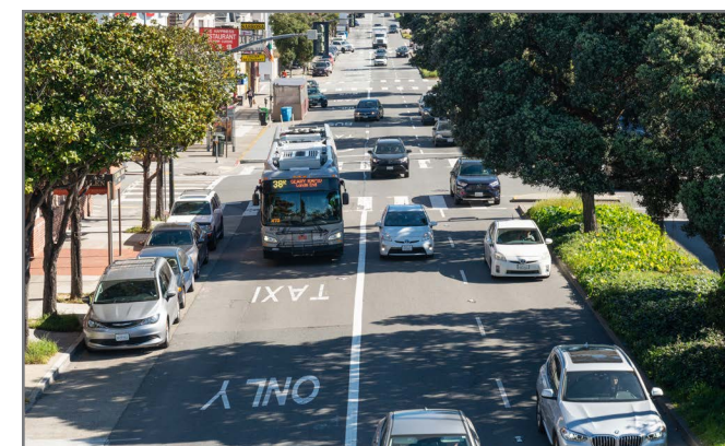
Quick-build transit lane in the Richmond: New transit lanes were installed as part of the Temporary Emergency Transit Lanes program and were later approved permanently.
