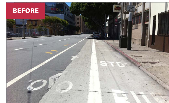
Otis Street at South Van Ness Avenue (before): The 14 Mission bus stop was located to the right of the bike lane, increasing the chance of conflicts, with no dedicated lane for buses.
