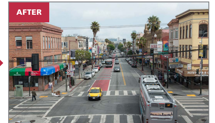
Mission Street at 20th Street (after): Removing a northbound lane and requiring northbound cars to turn right every few blocks reduced transit delay, while preserving most parking for businesses and making room for a southbound transit lane.
