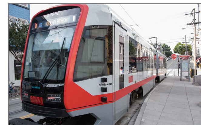
Transit bulb on Carl Street: Transit bulbs on Carl Street make it easier and safer for riders to board.
