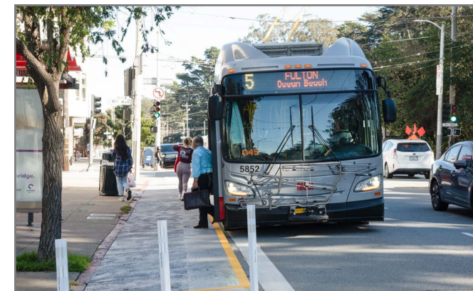
Temporary transit bulb on Fulton Street: Quick-build transit bulbs made of wood were installed on Fulton Street at 6th and 8th avenues. These will soon be replaced by concrete bulbs.
