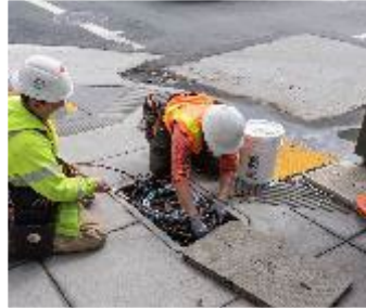
Existing Electrical Power
