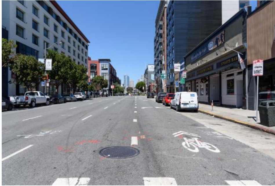
Existing sharrows on 3rd Street between King Street and Townsend Street
